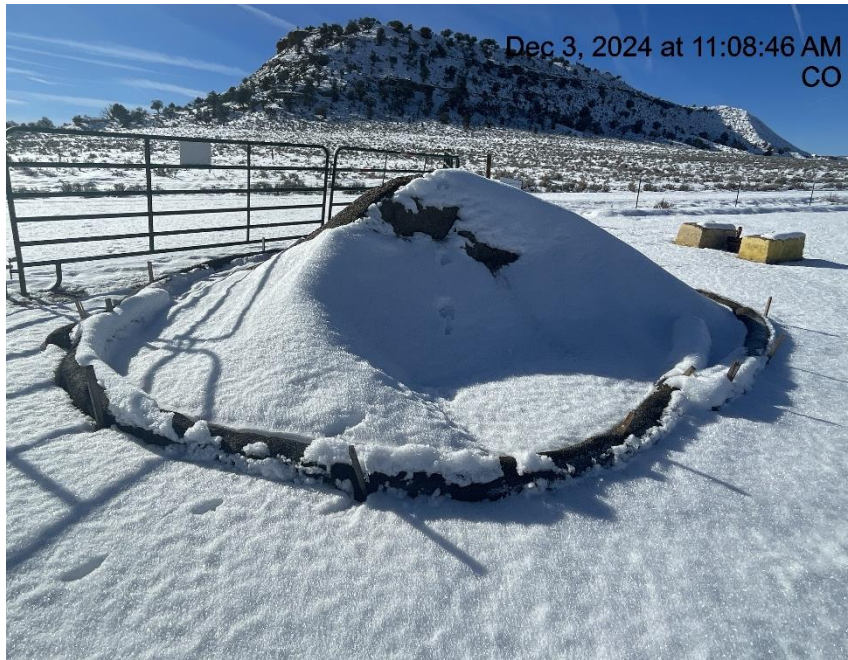
Photo # 2034 Stockpiled soils with BMP's
