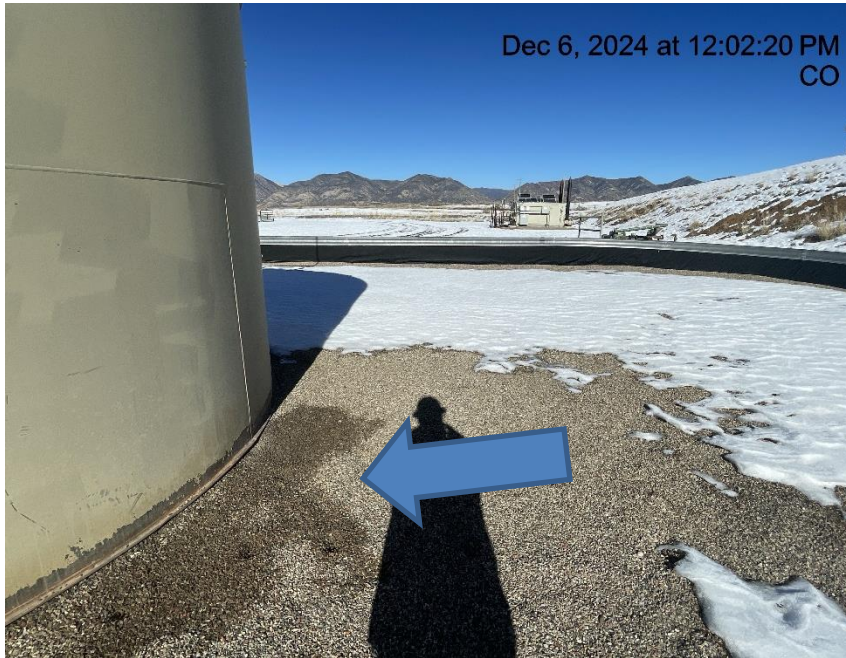
Photo # 2489 Staining in secondary containment
