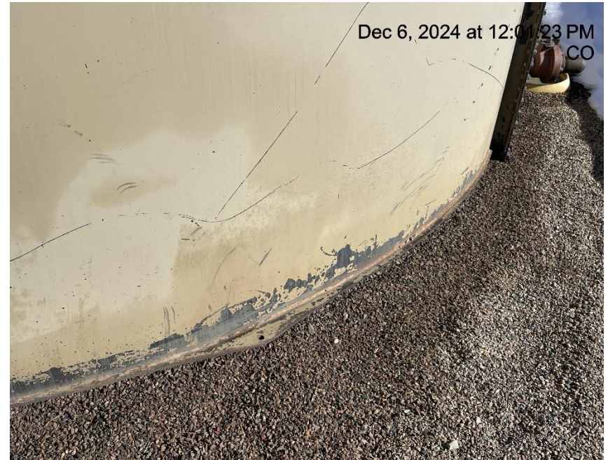
Photo # 2490 Staining in secondary containment
