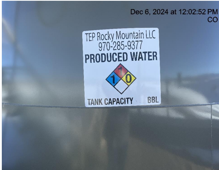
Photo # 2491 Tank capacity faded & illegible
