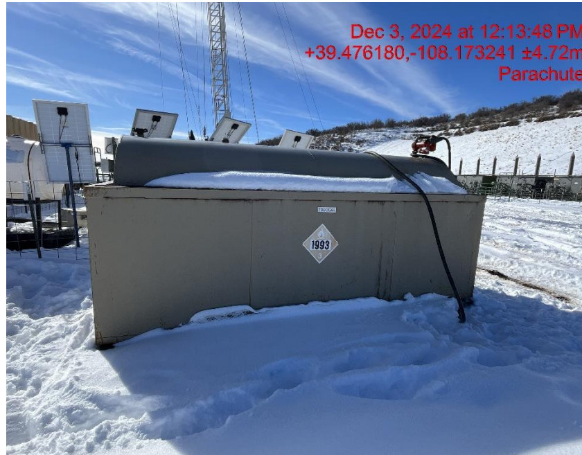
Photo # 0164 Diesel tank not properly labeled, missing required information
