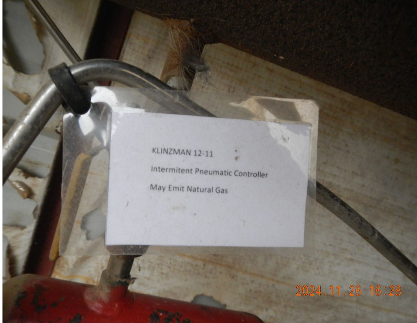
5. Equipment ID tag on controller used to identify well associated with equipment.
