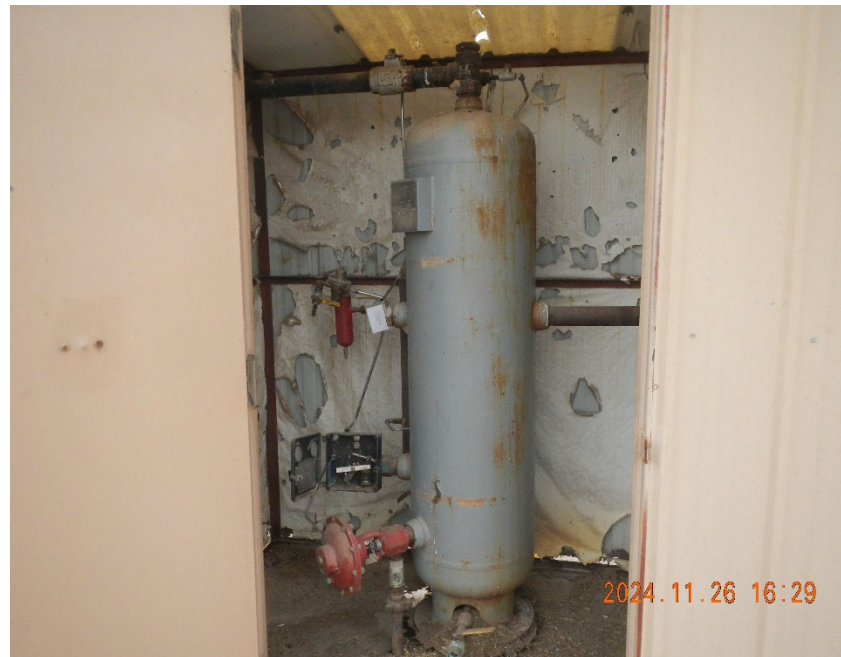
4. Vertical separator inside separator shed.
