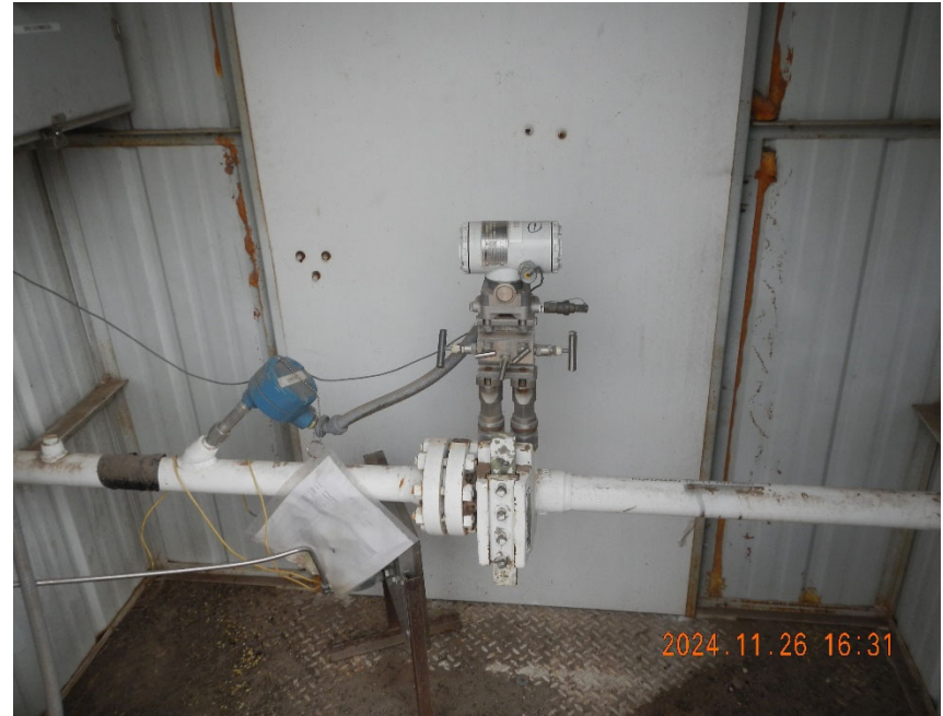
8. Gas meter inside meter shed.
