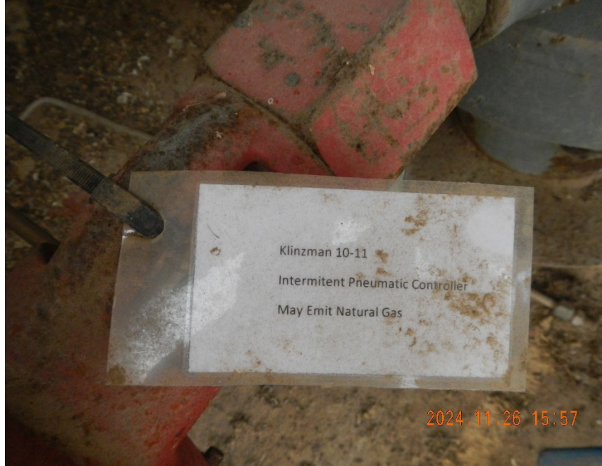
7. Equipment ID tag on controller used to identify well associated with equipment.
