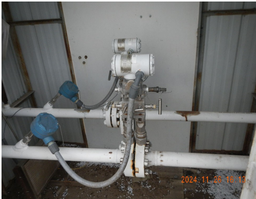
5. Gas meter inside remote meter shed.
