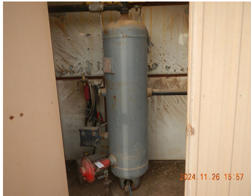
6. Vertical separator inside remote separator shed.
