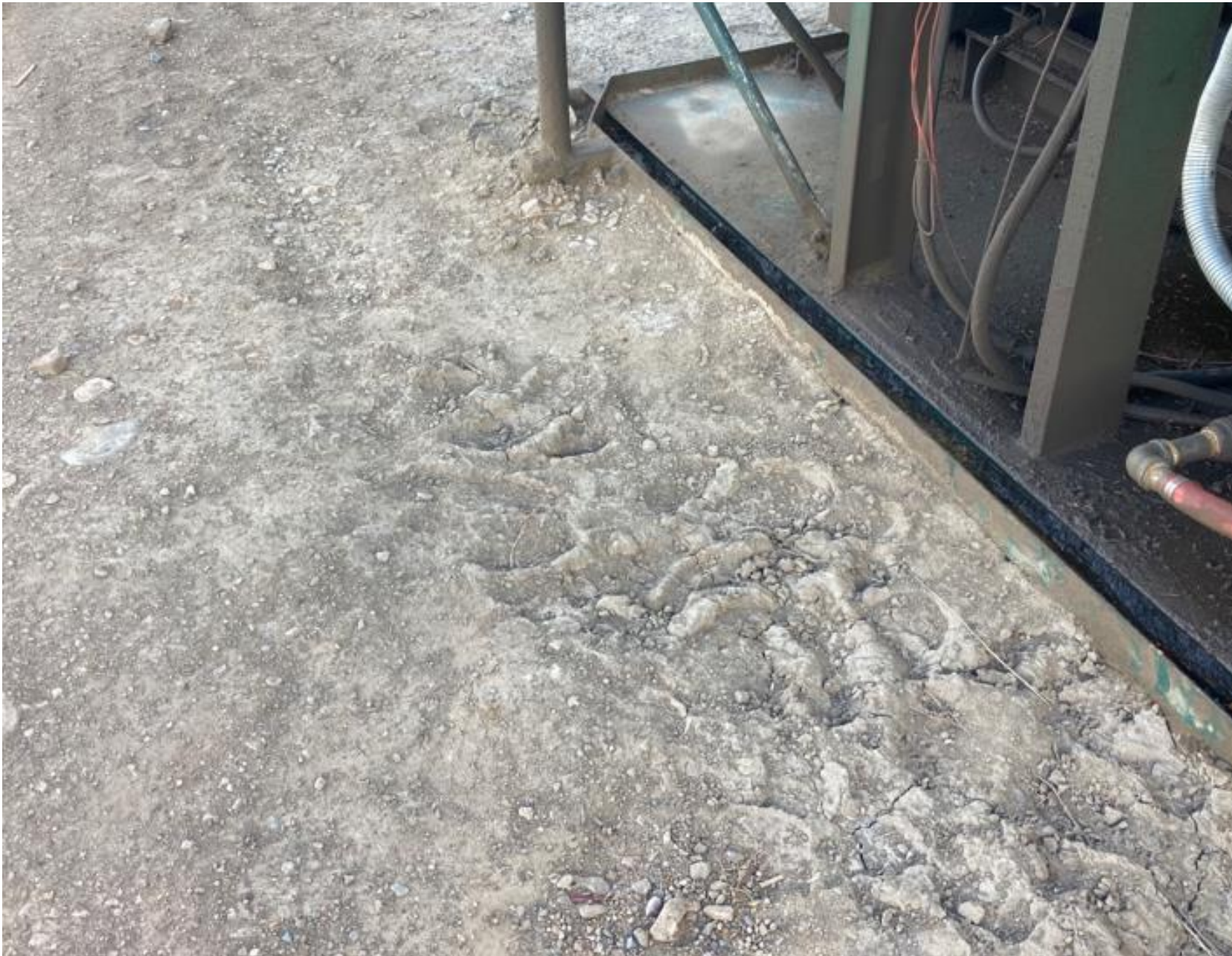
PHOTO 1: THE ENGINE HAS RECEIVED MECHANICAL MAINTENANCE AND THE OIL LEAK STOPPED. THE SKID HAS BEEN CLEANED OF ALL OILY FLUIDS. THE IMPACTED SOIL AROUND THE SKID HAS BEEN REMOVED AND REPLACED WITH FRESH MATERIAL.
