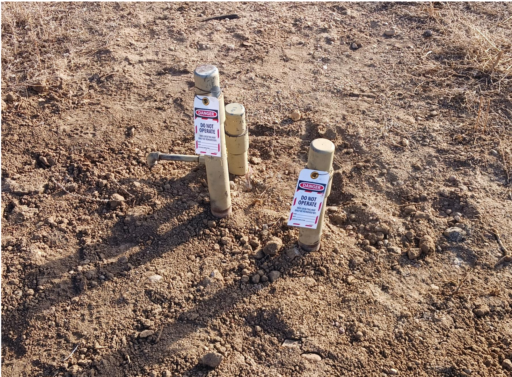
Figure #1 Weeds and trash have been removed. Risers have been LOTO.
