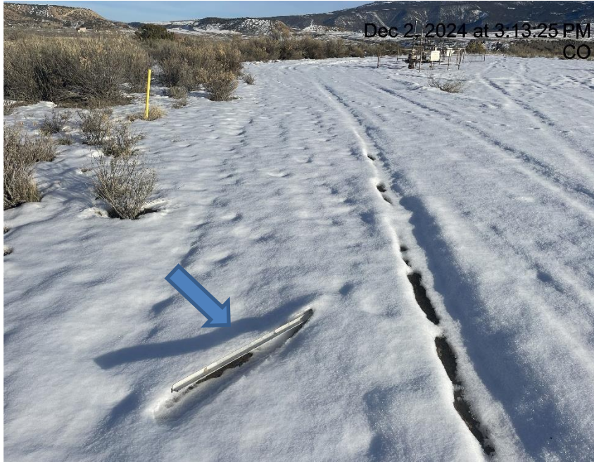
Photo # 1983 Improperly marked deadman
