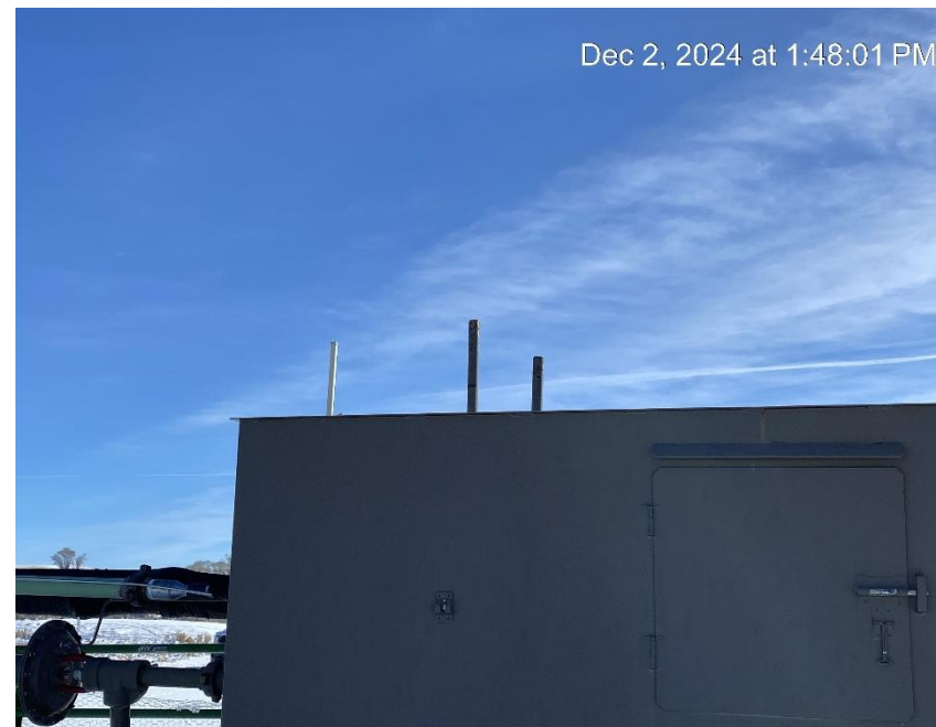
Vent risers missing caps
