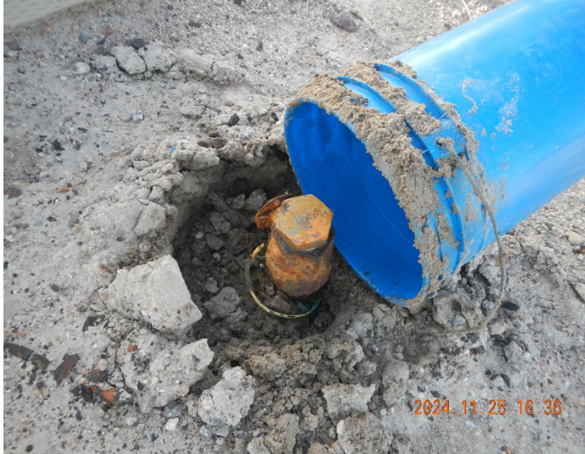
3. Flowline riser at wellhead where water leg was disconnected.
