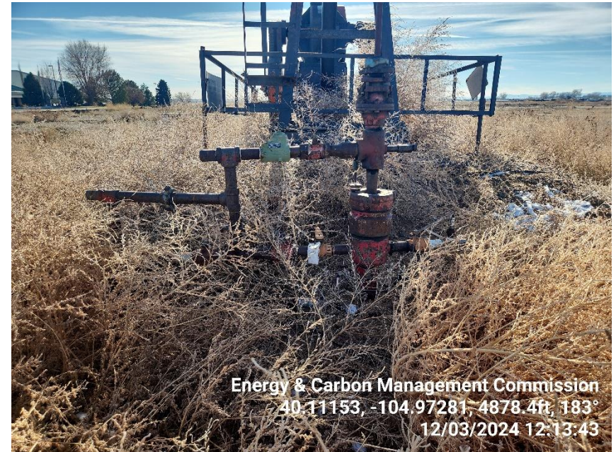
Photo 2 Wellhead over run with dead vegetation.
