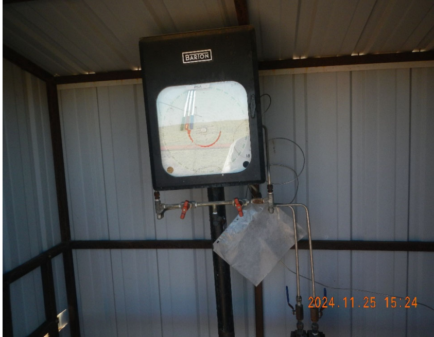
5. Gas meter inside meter shed.
