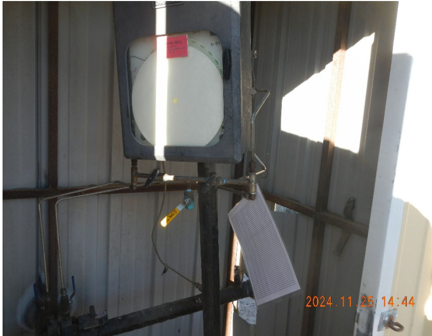
3. Gas meter inside meter shed.
