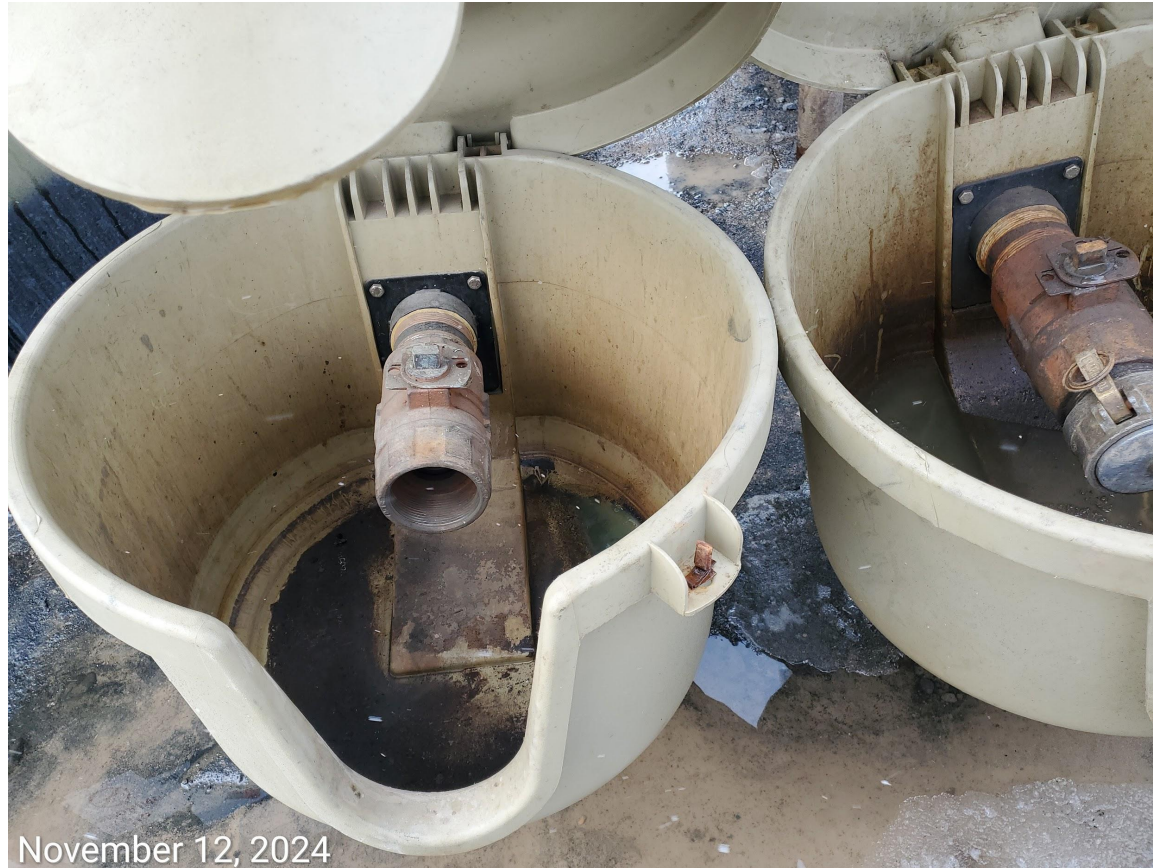
Photo 2: Lines at tanks missing cap/plug.
