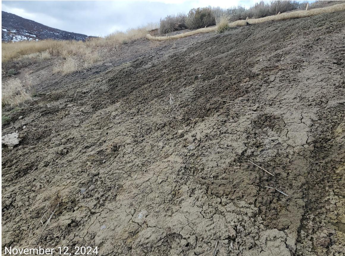
**Photo 3:** See comments under photo 2. Erosion degradation is recurring; unable to find evidence of seeding; BMPs to stabilize soils remain missing/insufficient.
