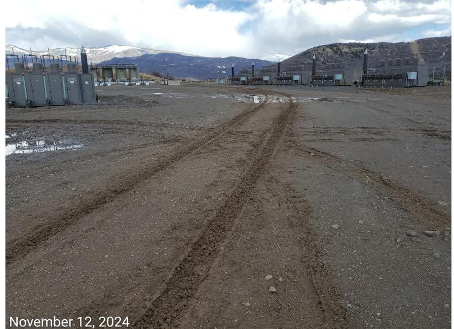
**Photo 1:** Photos examples showing that the BMPs to stabilize the working pad surface, as well as to minimize erosion, degradation, and sediment transport are in disrepair; tracking/degradation apparent.
