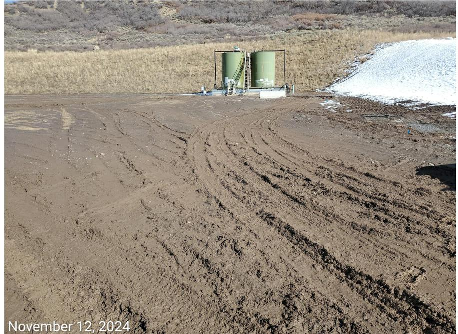
**Photo 2:** Photos 2-4 examples showing that the working pad surface lacks stabilization; BMPs to stabilize the pad, as well as to minimize erosion, degradation, and sediment transport have not been maintained in proper functioning condition.
