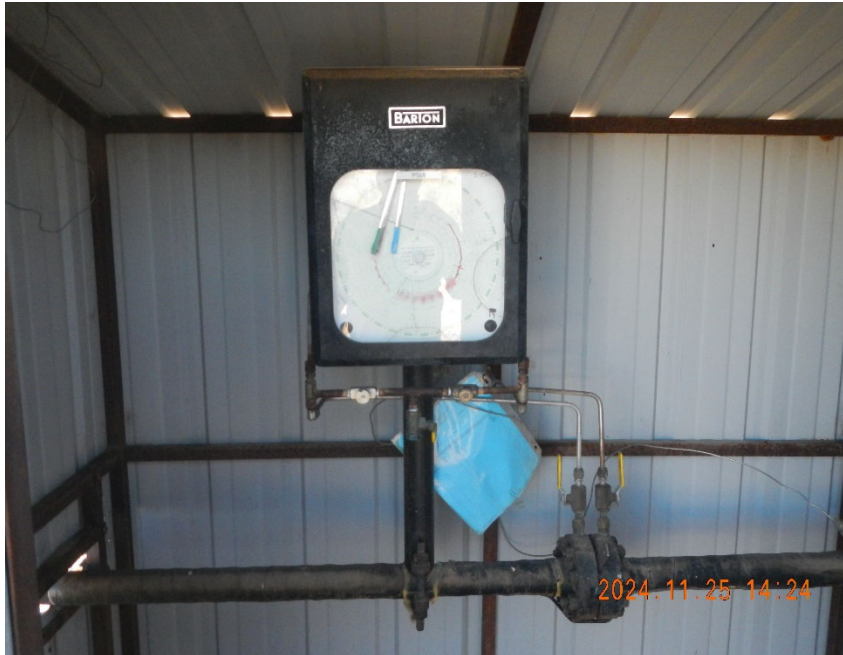
7. Shared gas meter inside meter shed.
