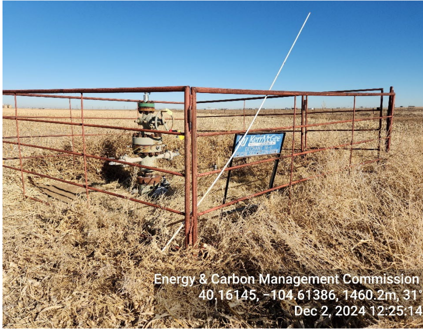
Photo 3: TA Wellhead; overgrown vegetation
