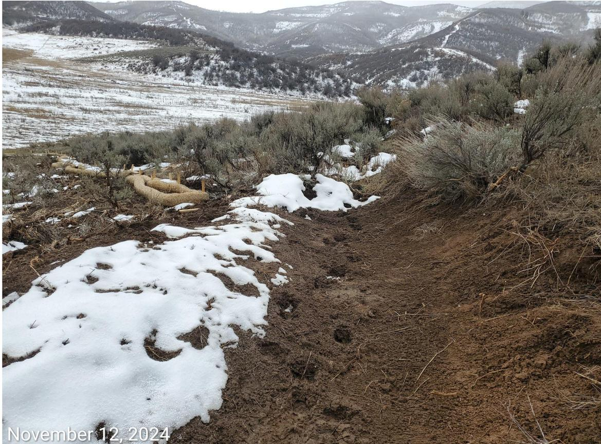
**Photo 12:** Photos taken from the diversion ditch on the west end of the Location, facing south. Photo shows BMP is incomplete and does not divert stormwater to the sediment trap on the southwest end of the Location per the Form 2A Layout drawing and SWMP. BMP currently missing a properly engineered outlet, such as a sediment trap with inlet/outlet protections, per good engineering practice.
