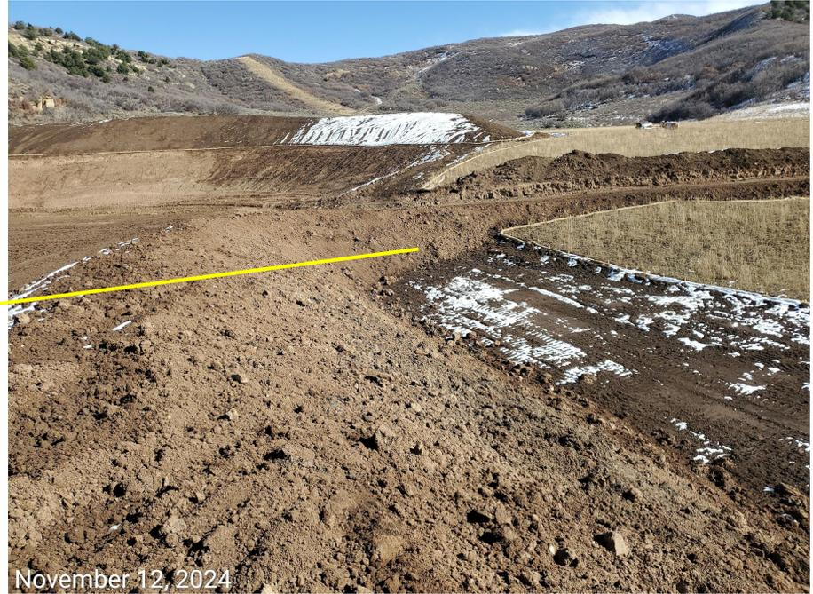
**Photo 14:** Photos taken from the fill slopes and Location entrance. Photos show BMPs to minimize erosion and degradation from the fill slopes are missing or insufficient; slopes currently bare unstabilized. Additionally, photos also show that the culvert/sediment trap/ditch have not been installed per the Form 2A SWMP and Layout drawing.
