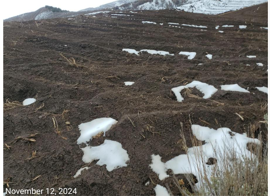
**Photo 5:** Photos taken from the topsoil stockpile on the east/northeast end of the Location. Soils are currently bare and at risk to wind and water erosion; BMPs to protect, as well as to minimize erosion and degradation are missing or insufficient.
