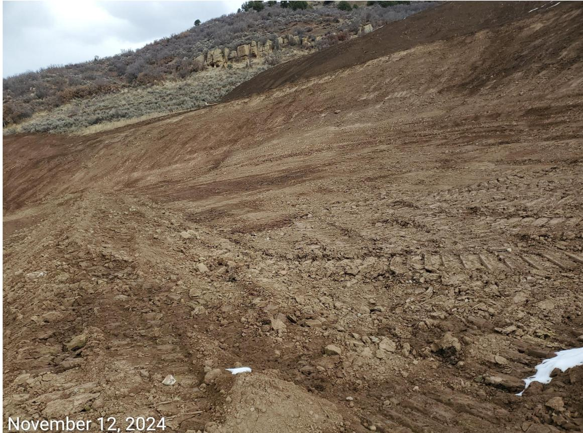
**Photo 4:** Photo taken from the east end of the Location. Photo shows cuttings trench constructed for disposal of drill cuttings. Trench requires permitting via Form 15.
