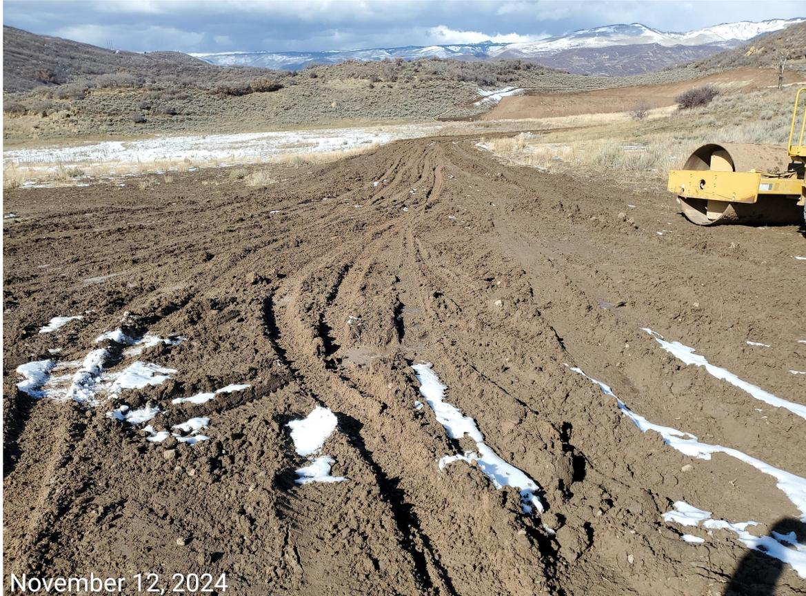
**Photo 19:** Photo example of tracking/stabilization issues observed on Location/Access road. BMPs to stabilize, as well as to minimize degradation and sediment transport are missing or insufficient.
