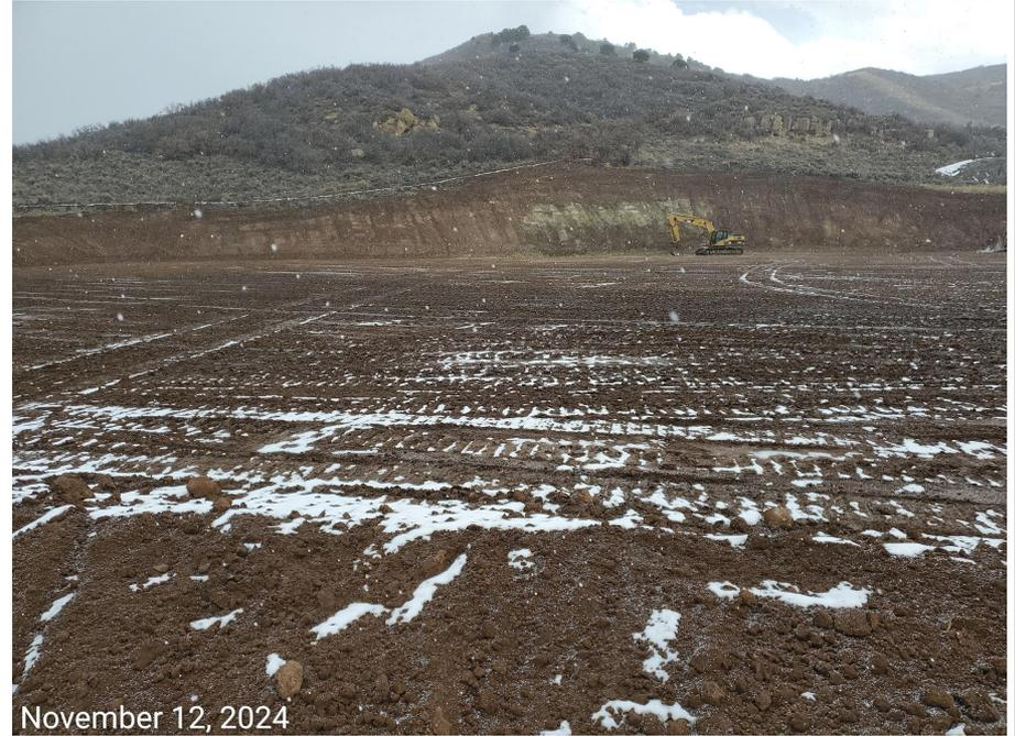
**Photo 9:** Photos 9-10 taken from the west end of the working pad surface. Photos provide an overview from north, northeast, southeast to south. Photos also show ditch along perimeter of the pad has not been installed.
