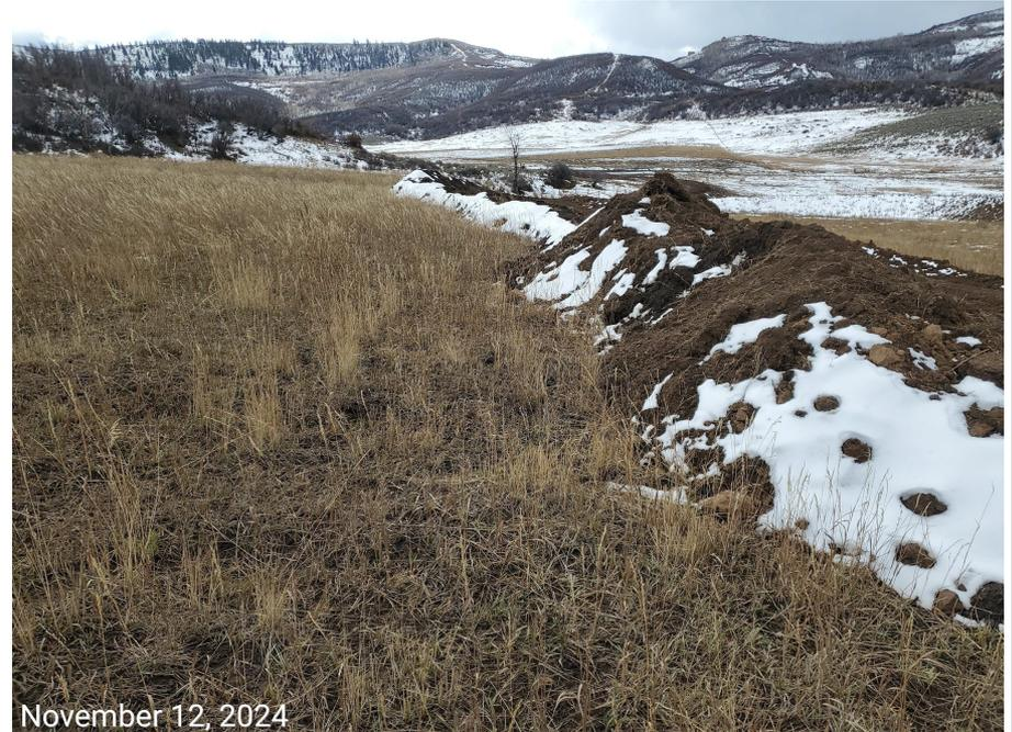
**Photo 6:** Photos taken from the topsoil stockpile along the access road. BMPs to minimize erosion, degradation and sediment transport are missing or insufficient.
