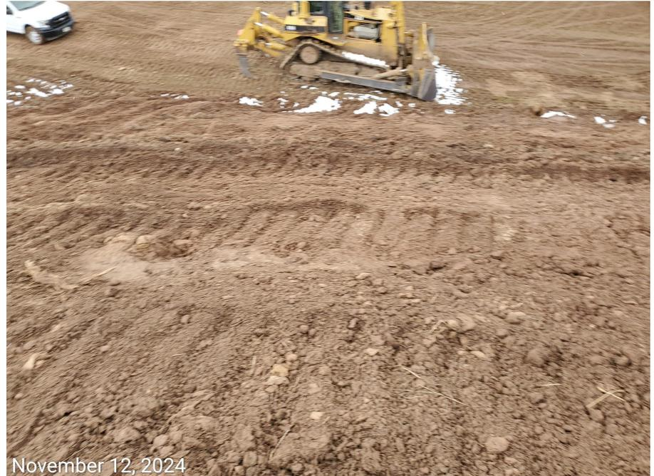
**Photo 8:** Photos taken from the cut slopes on the east end of the Location. Photos examples showing BMPs to minimize erosion and degradation from the cut slopes are missing or insufficient; slopes currently bare unstabilized.
