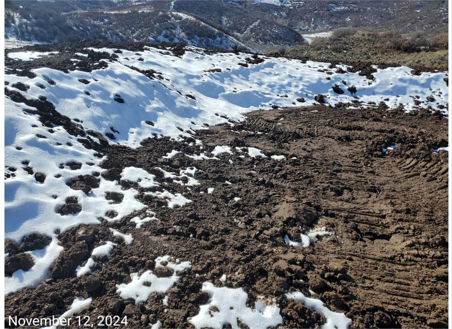
**Photo 15:** Photos taken from the southwest corner of the working pad surface. Photo shows slope drain has not been installed per the Form 2A SWMP and Layout drawing. Photos also examples showing pad surface lacks stabilization.
