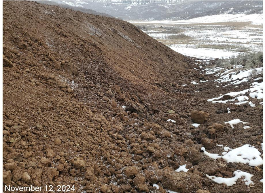
**Photo 11:** Photos taken from the west end of the Location, facing south. Photos examples showing BMPs to minimize erosion and degradation at the fill slopes are missing or insufficient; slopes currently bare unstabilized. Photo left also shows BMPs per the SWMP (Slope drain) have not been installed.
