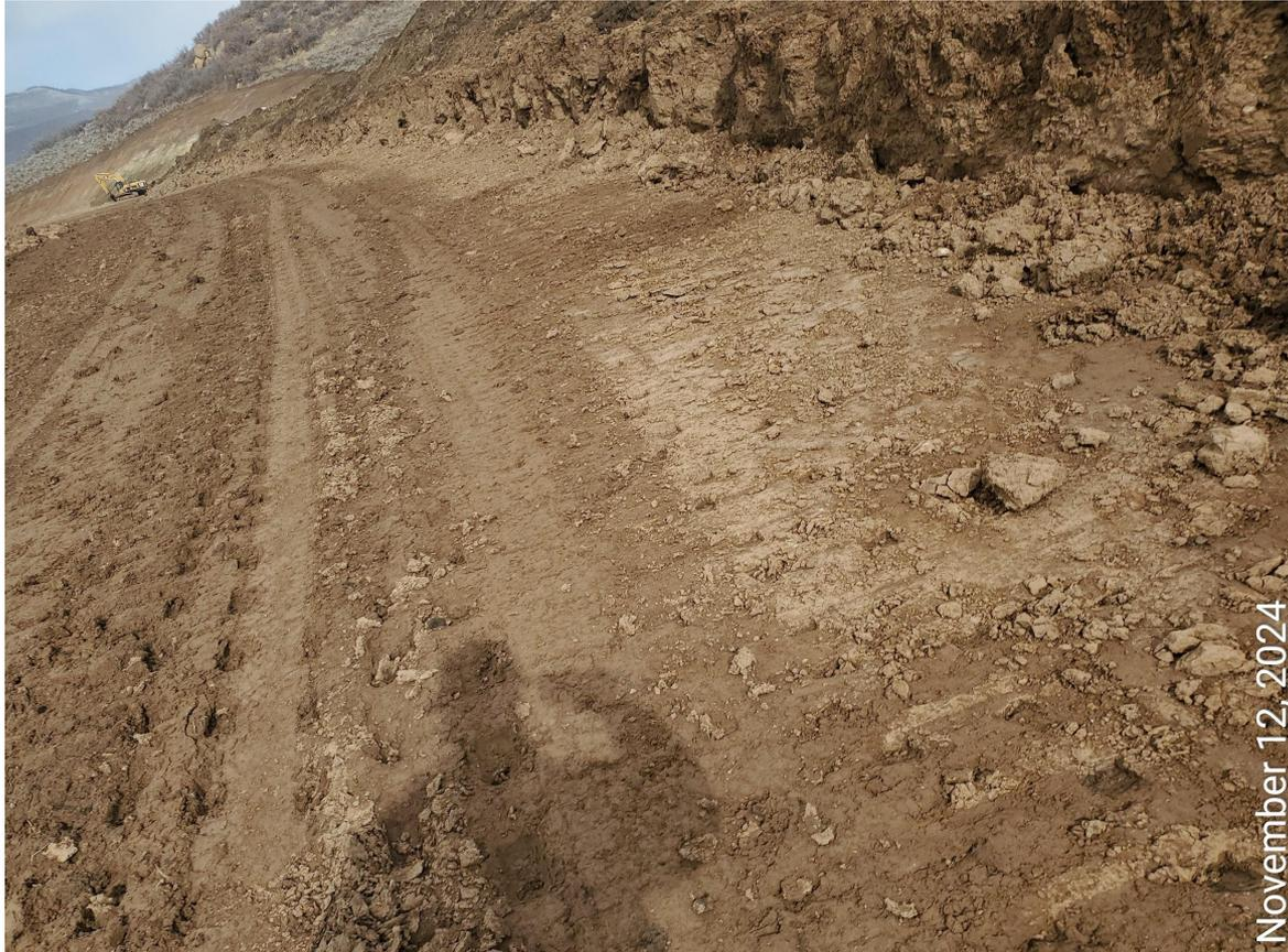
**Photo 18:** Ditch has not been constructed along access road. Culvert also missing along access road per the Form 2A SWMP and Layout drawing.
