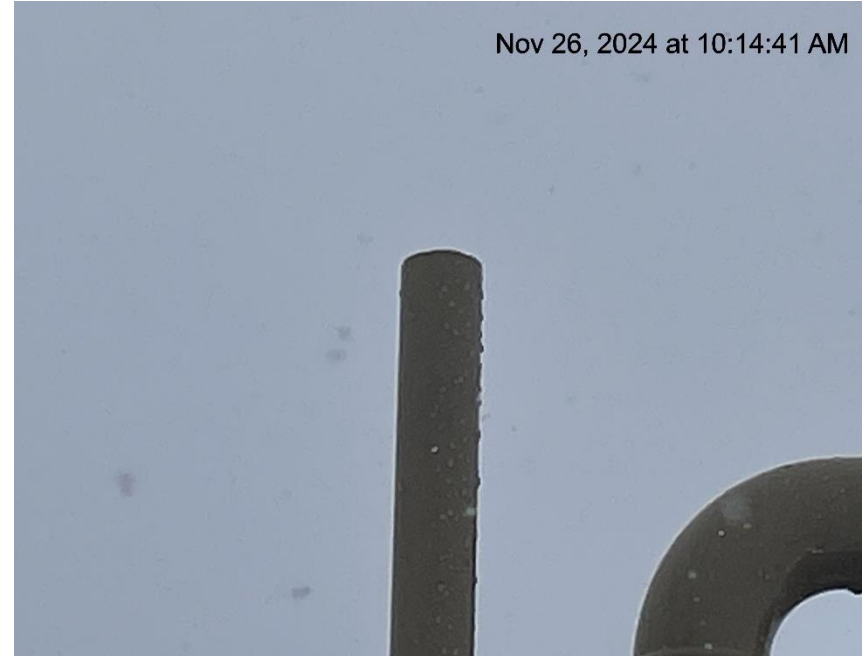
Photo # 1281 PRV vent line does not comply with CECMC pressure safety device rules
