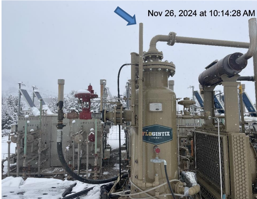
Photo # 1280 PRV vent line does not comply with CECMC pressure safety device rules
