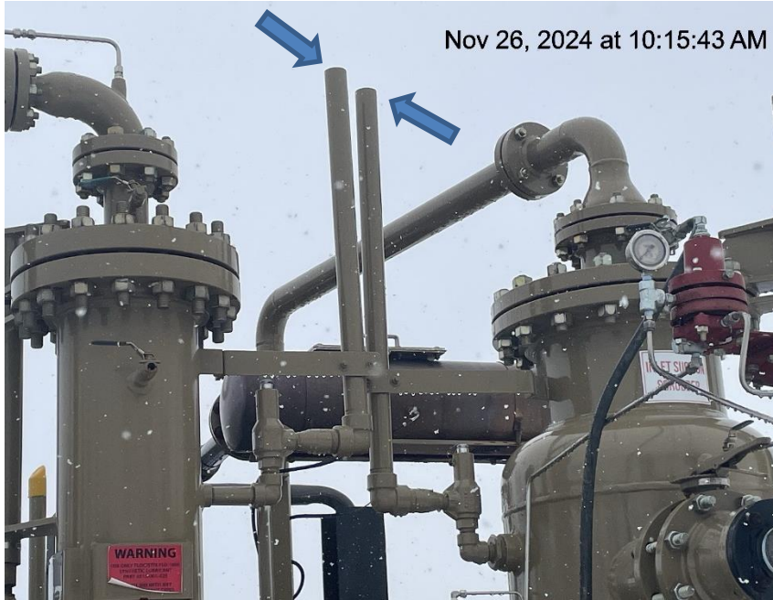
Photo # 1282 PRV vent lines do not comply with CECMC pressure safety device rules
