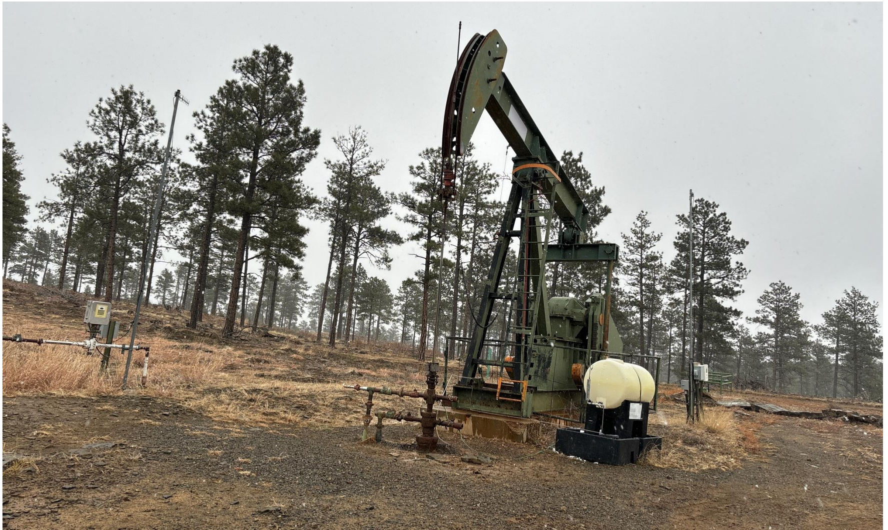
PHOTO 3: WELLHEAD AND EQUIPMENT.
