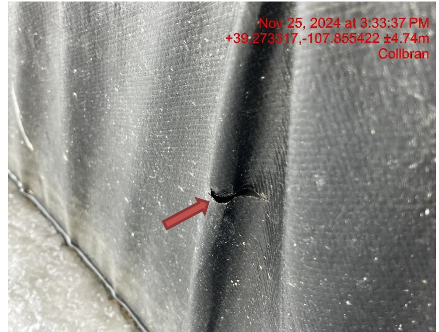
Photo # 9944 Multiple holes in secondary containment liner/liner needs maintenance
