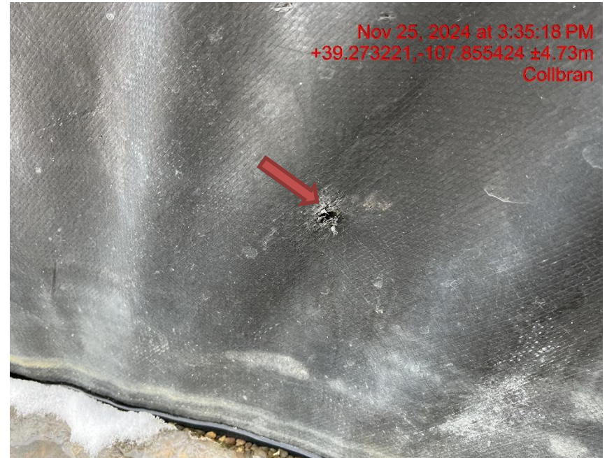
Photo # 9948 Multiple holes in secondary containment liner/liner needs maintenance
