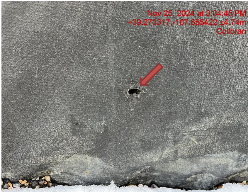
Photo # 9947 Multiple holes in secondary containment liner/liner needs maintenance
