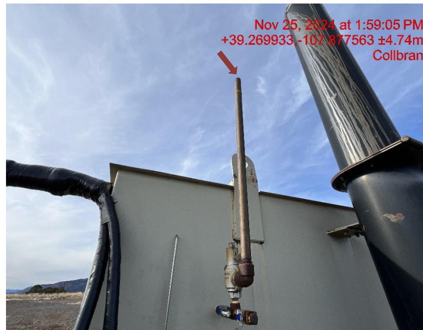
Photo # 9876 PRV vent line does not comply with CECMC pressure safety device rules
