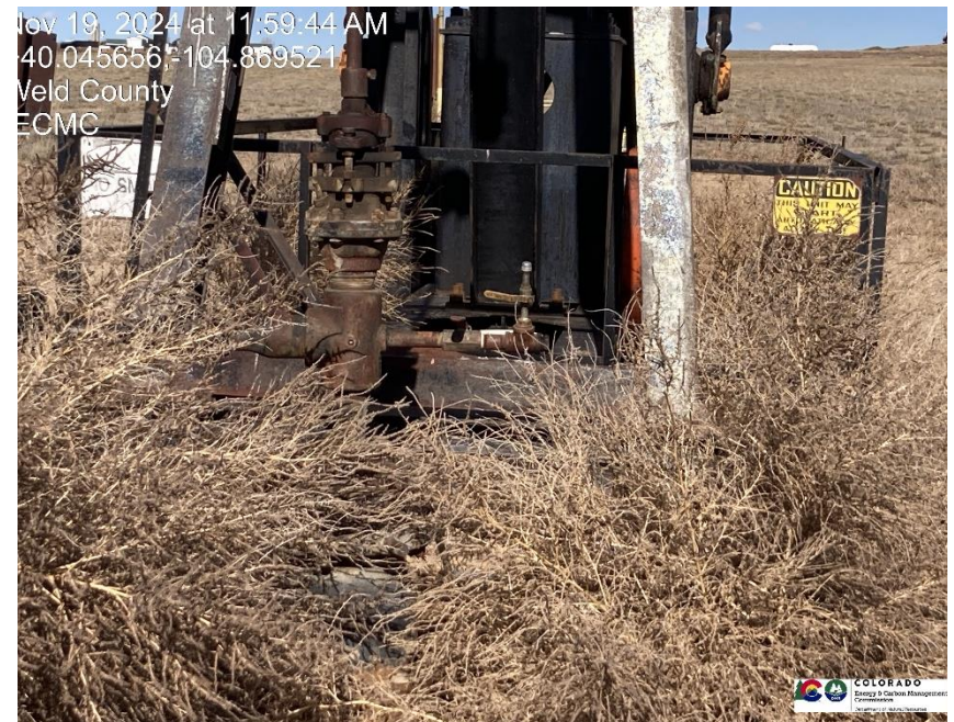
Pic 2 Wellhead sign needs to be put back up
