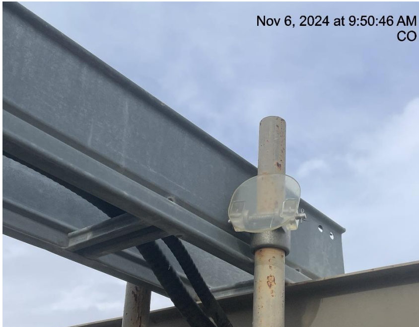
Photo # 9091 From inspection 708904991 conducted on 11/06/2024 PRV vent line does not comply with CECMC pressure safety device rules
