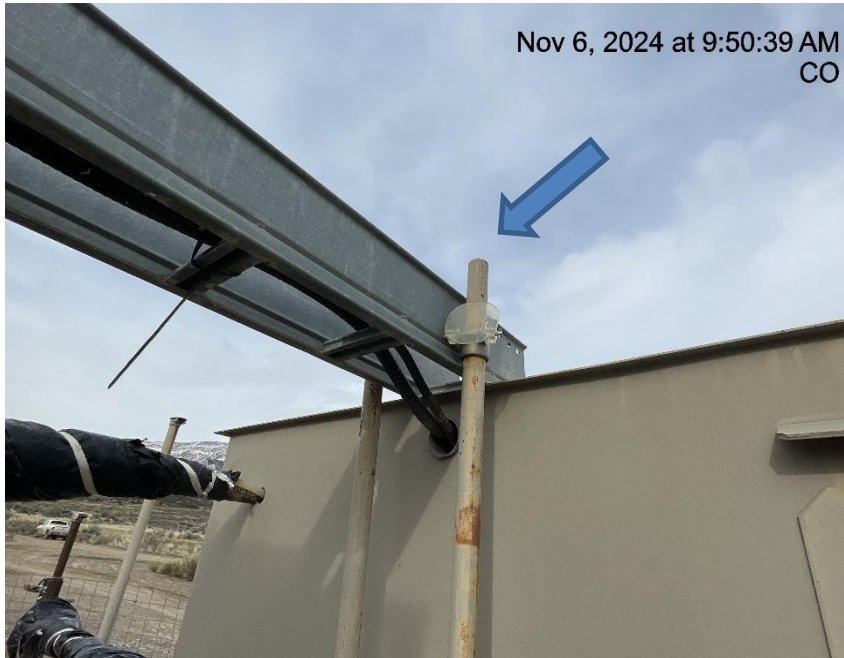
Photo # 9090 From inspection 708904991 conducted on 11/06/2024 PRV vent line does not comply with CECMC pressure safety device rules
