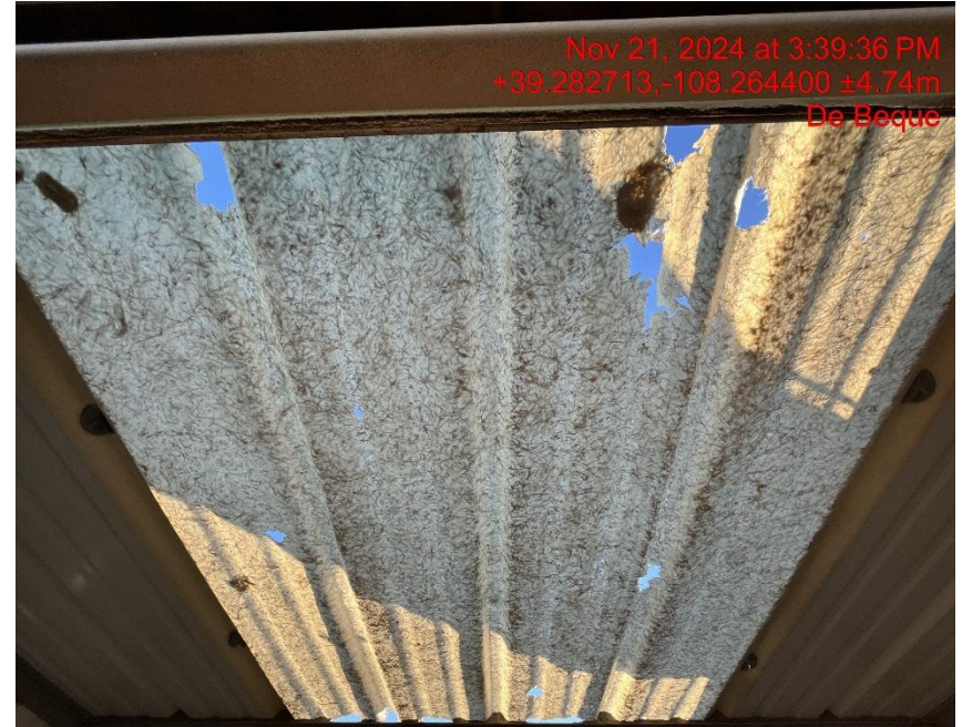
Photo # 9744 Gas meter building roof paneling is damaged/wildlife hazard available for entry by wildlife
