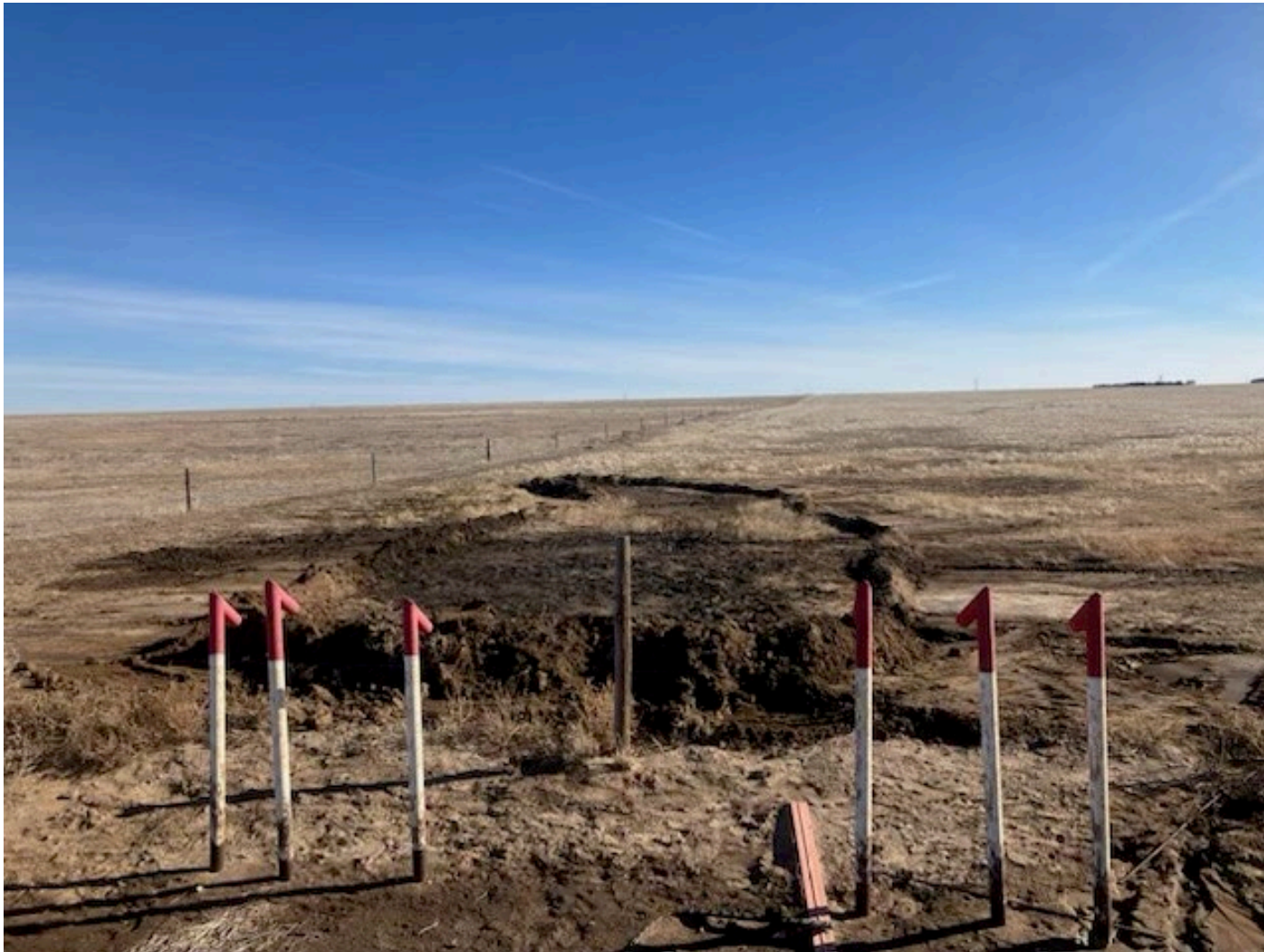
Containment berms around release point
