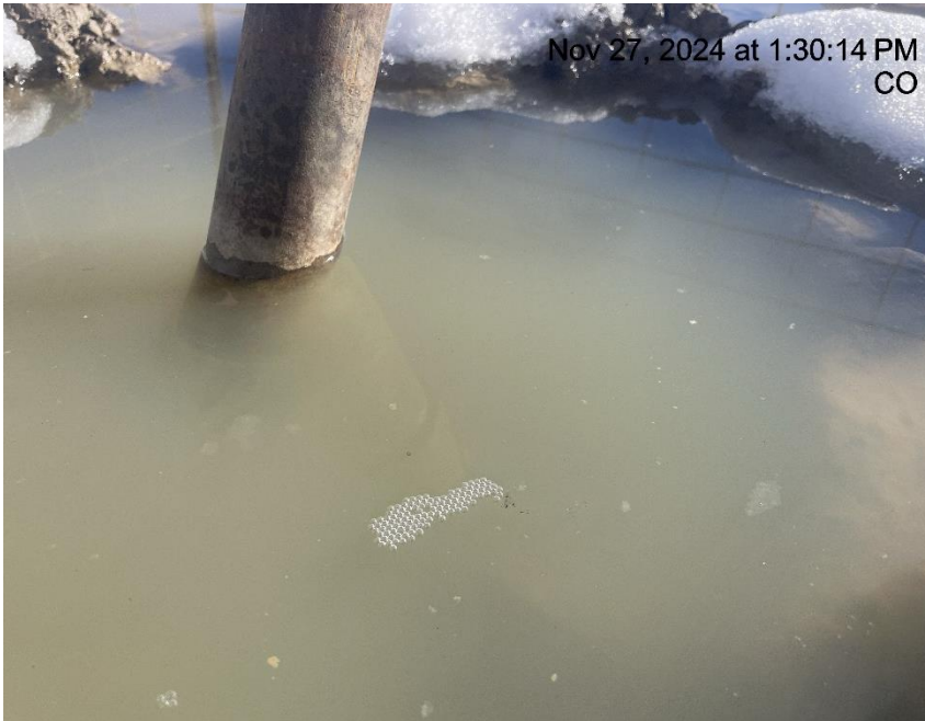
Photo # 1606 Mechanical Condition - possible bradenhead leak on the RMV 33-20 well
