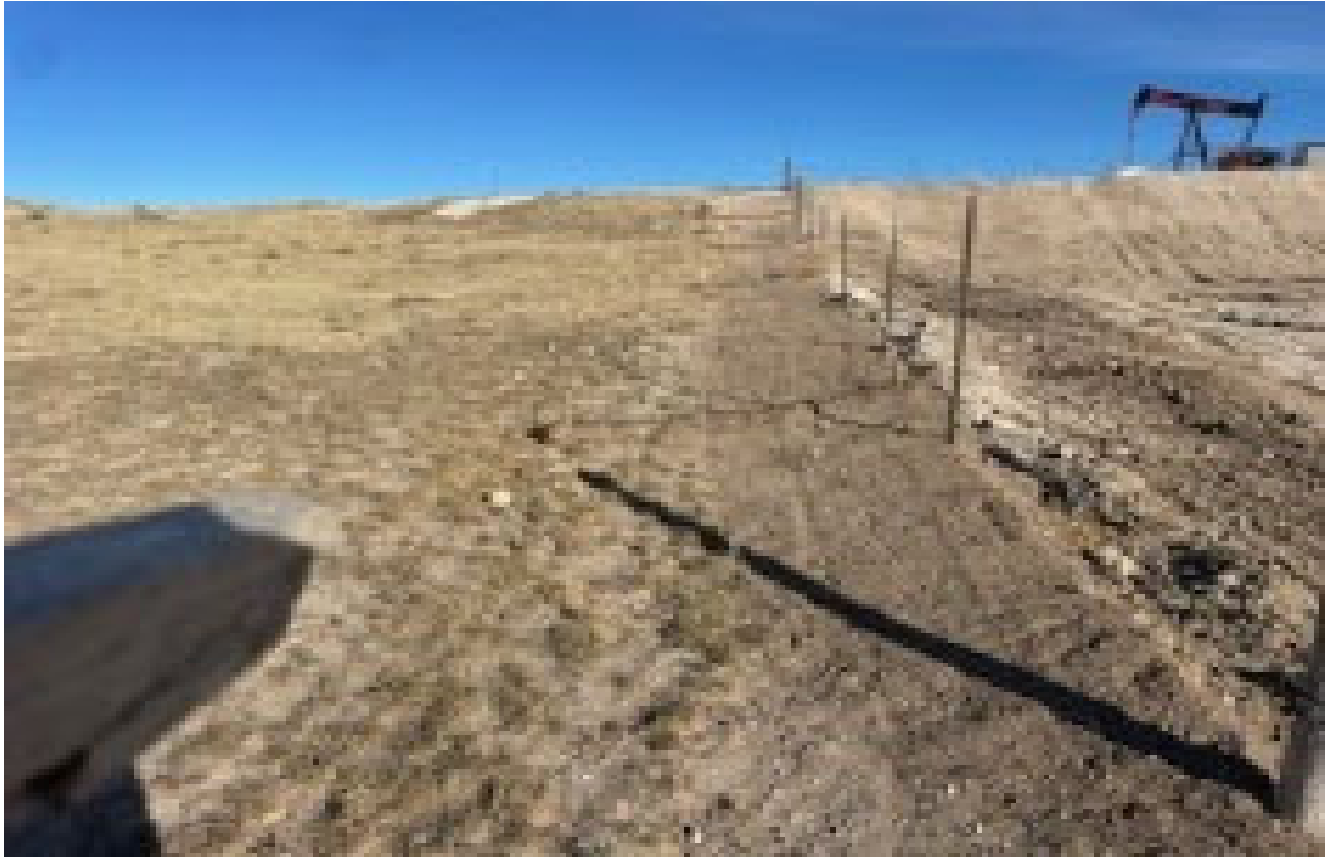
Straw Wattles installed on North end of excavation
