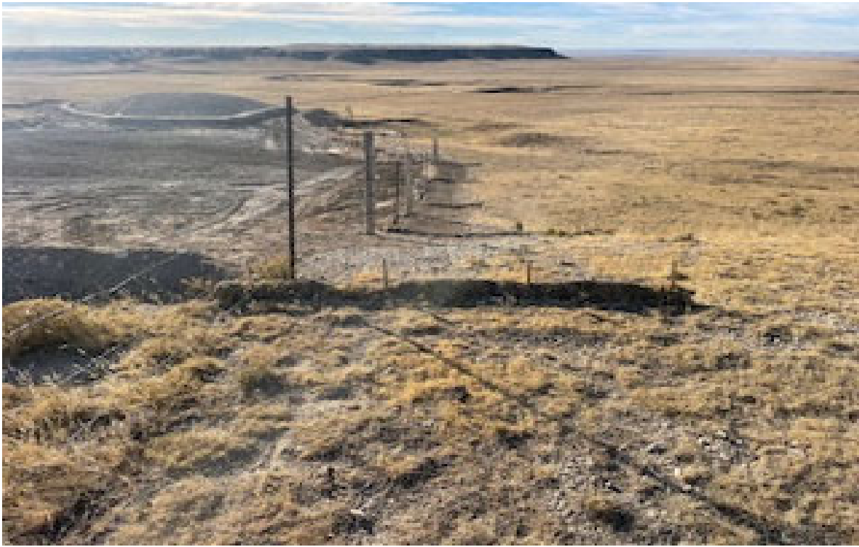
Straw Wattles installed on North end of excavation, trenched and backfilled
