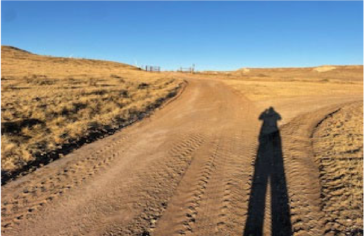
Access Road Graded looking towards entrance gate
