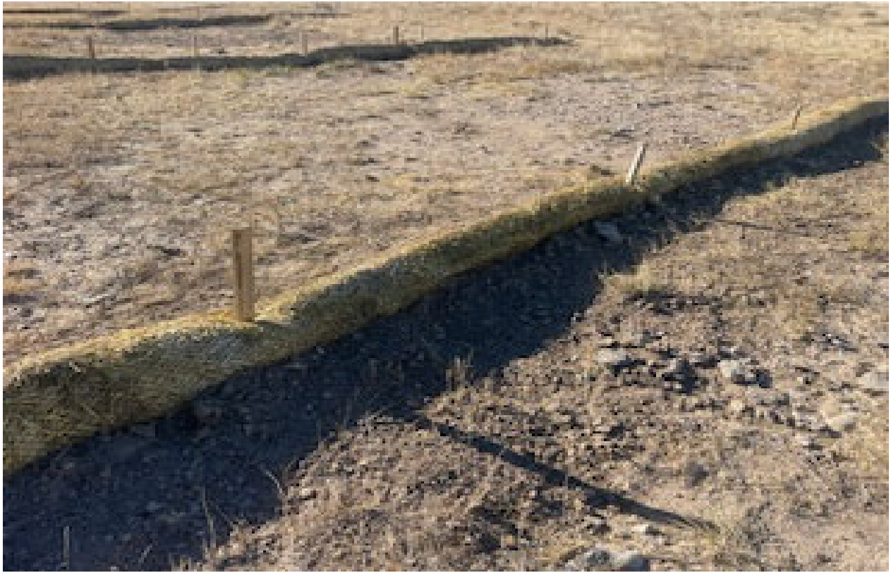
Straw Wattles South of old Separator Area, trenched and backfilled
