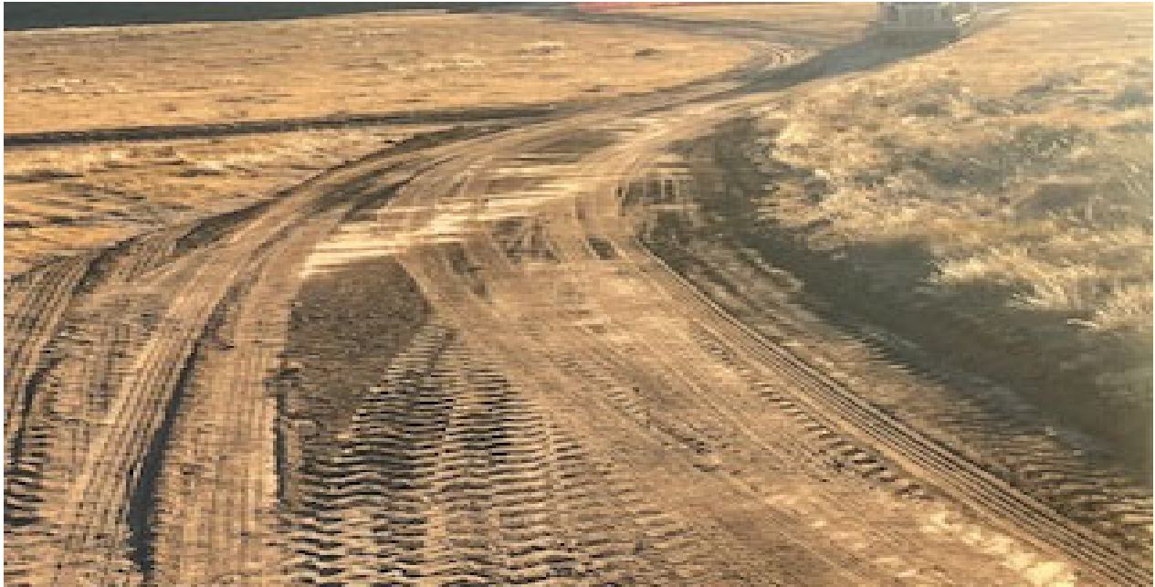
Access Road Graded fixed storm water erosion
