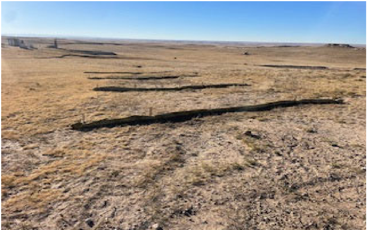
Straw Wattles re-installed South of old Separator Area, trenched and backfilled
