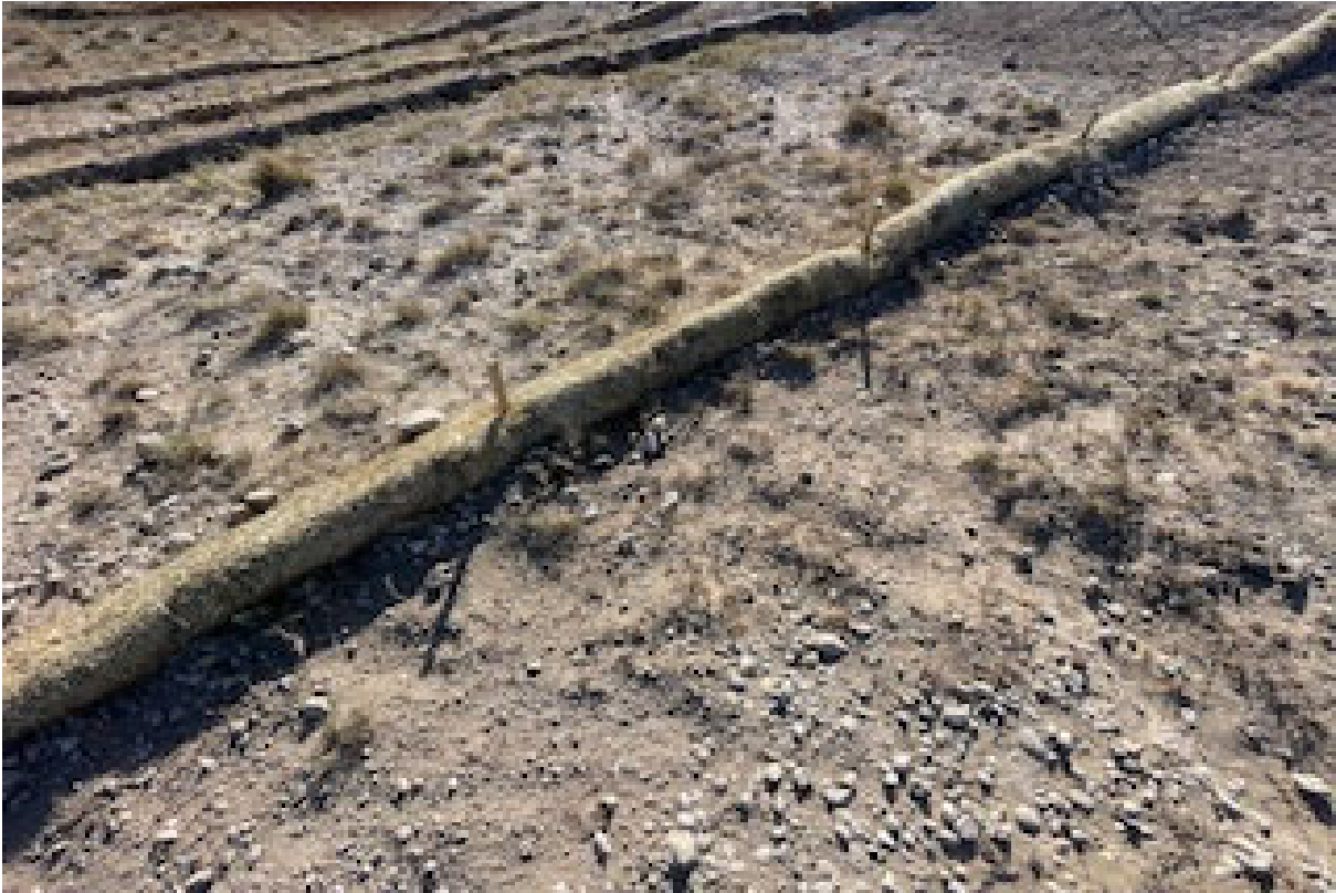
Straw Wattles installed South of Pump Jack, trenched and backfilled
