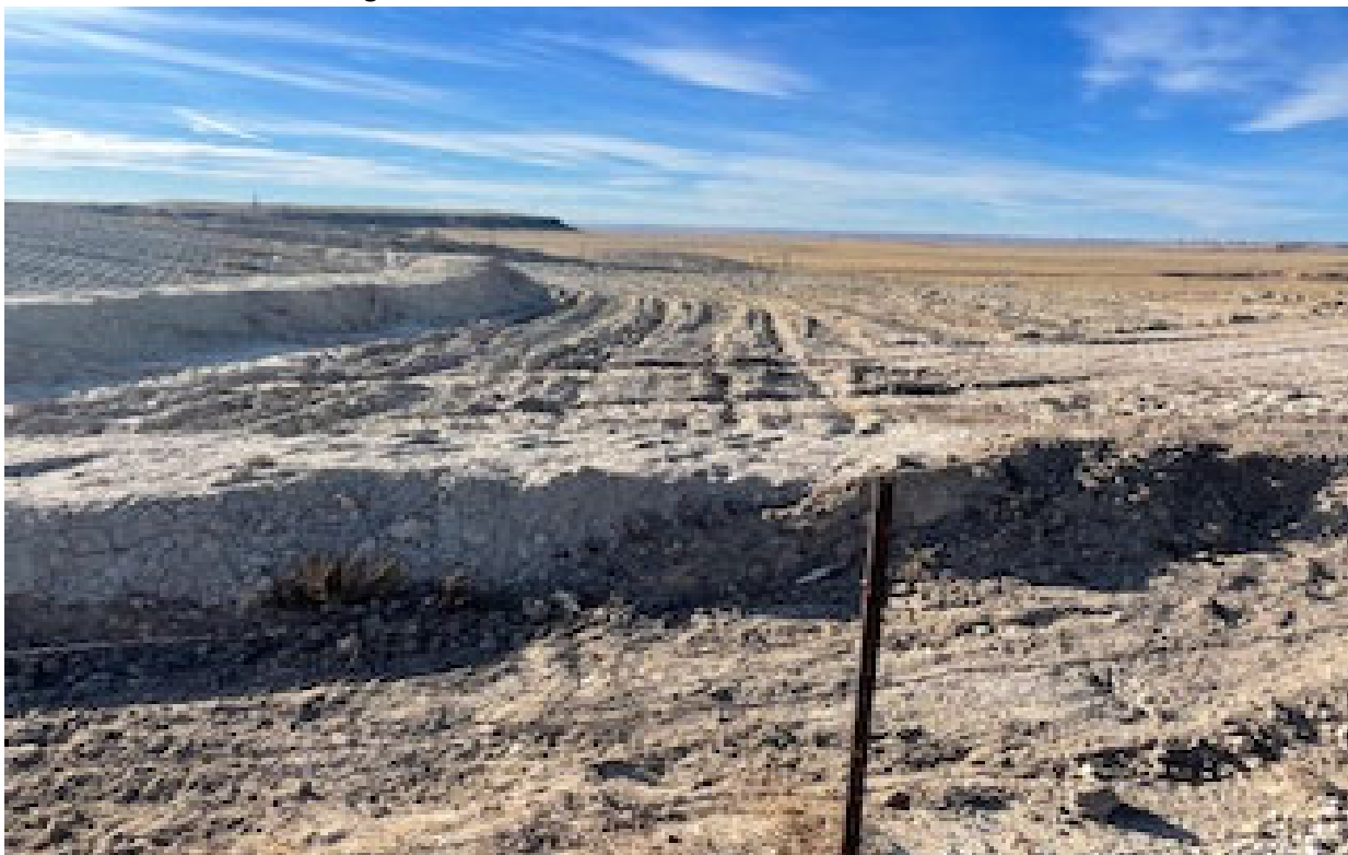
Looking from Southeast corner to the West across excavation
