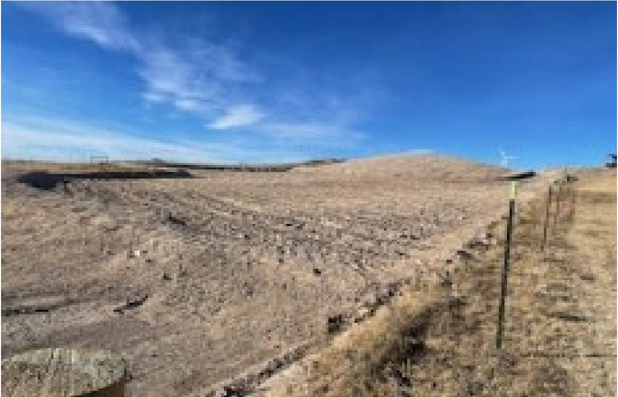
Southeast corner of excavation looking North
