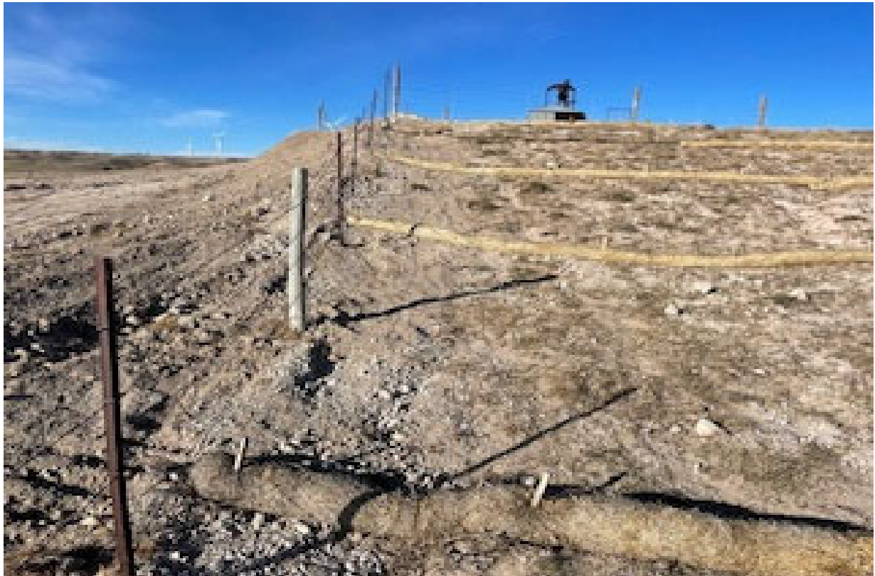
Straw Wattles installed and Storm water erosion fixed
