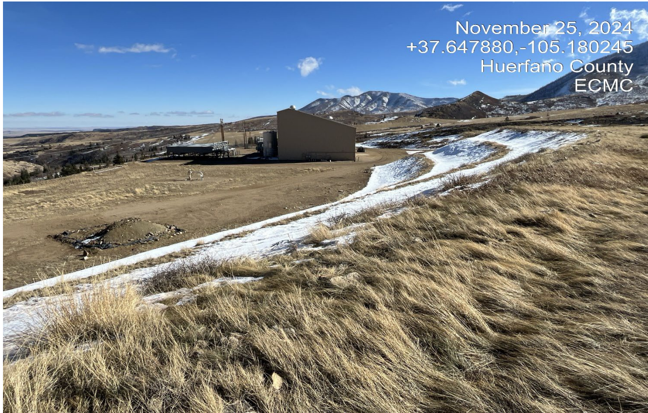
Photo 4. Facing southeast along the fill slope which will need to be partly recontoured. There are active wells that remain on the lower pad and far southeast side.
