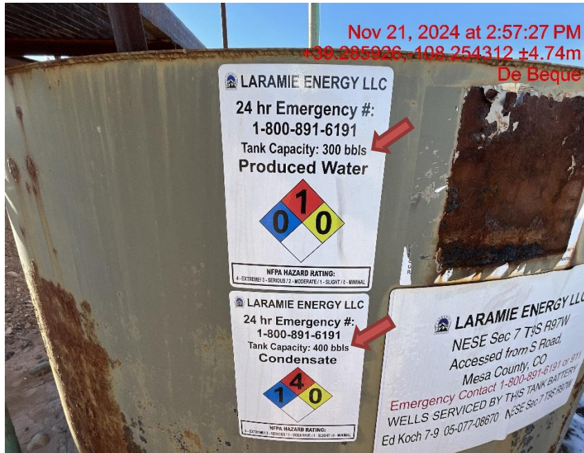
Photo # 9704 Tank labels have conflicting capacity information
