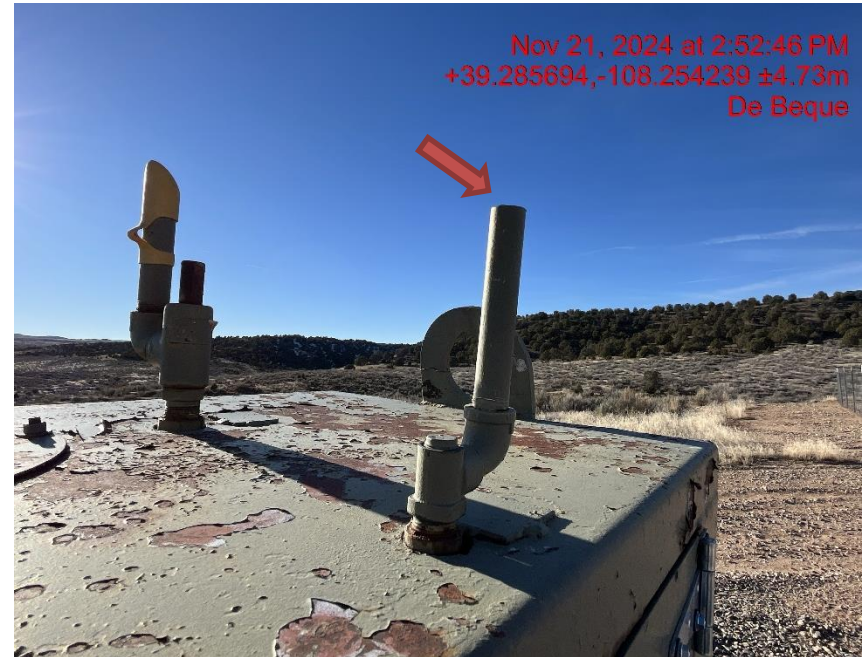
Photo # 9698 PRV vent line does not comply with CECMC pressure safety device rules
