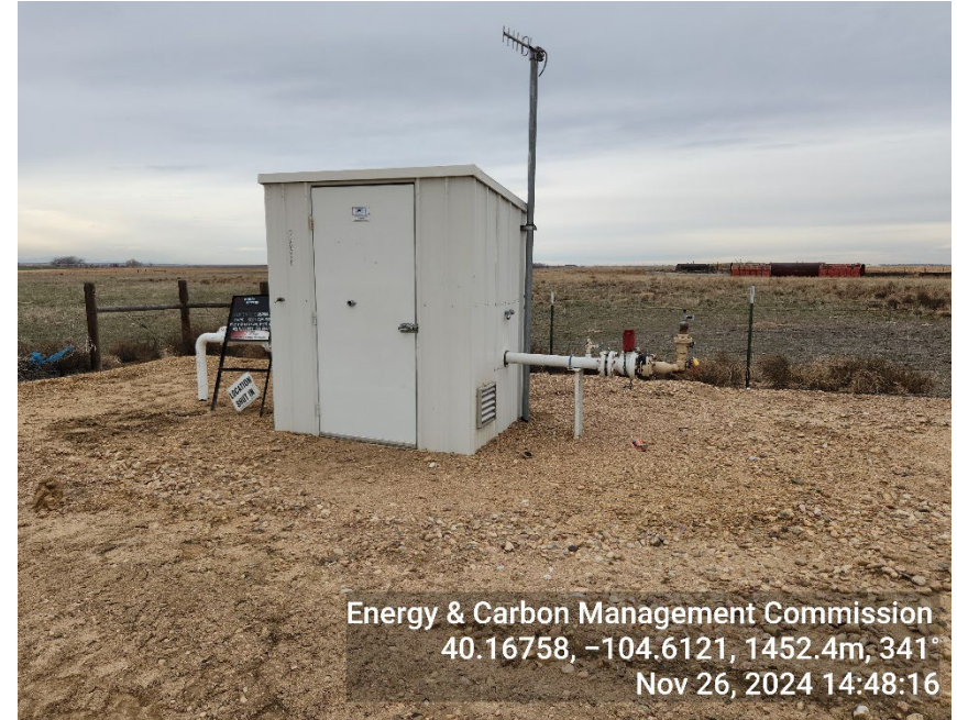
Photo 2: Unused/disconnected gas meter.
