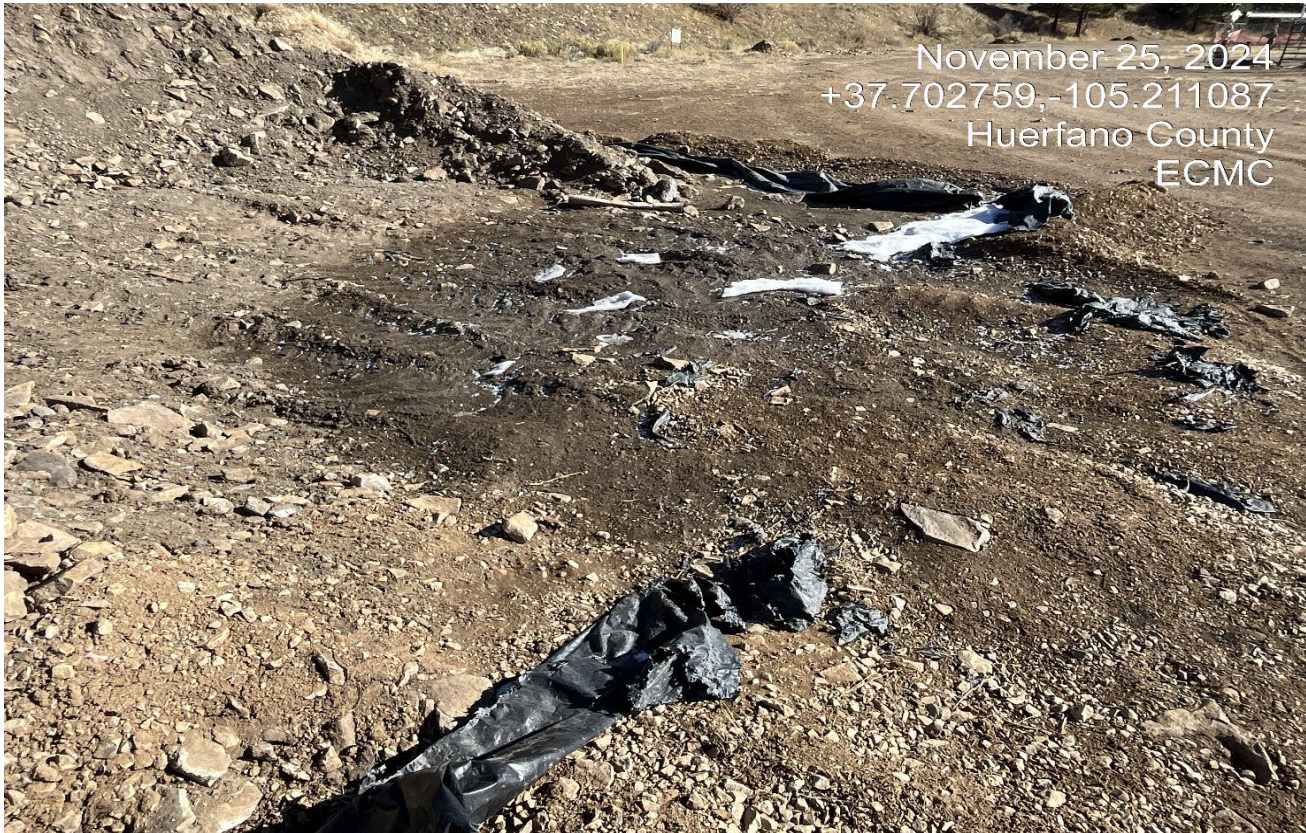
Photo 11. The waste material is contained and the liner is torn.
