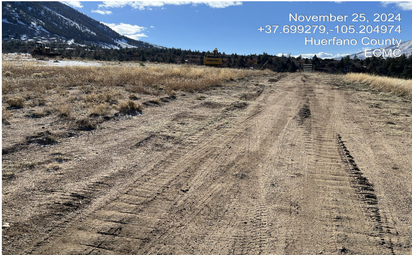
Photo 1. Facing south toward the access road.. The access road will need to be decompacted and reclaimed.
