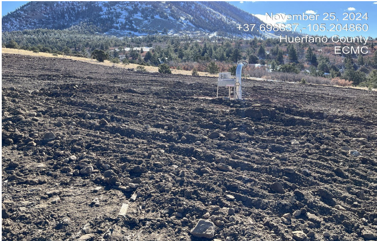
Photo 4. There is still a pipeline riser that remains at enter of the location that needs to be removed per the Rules.
