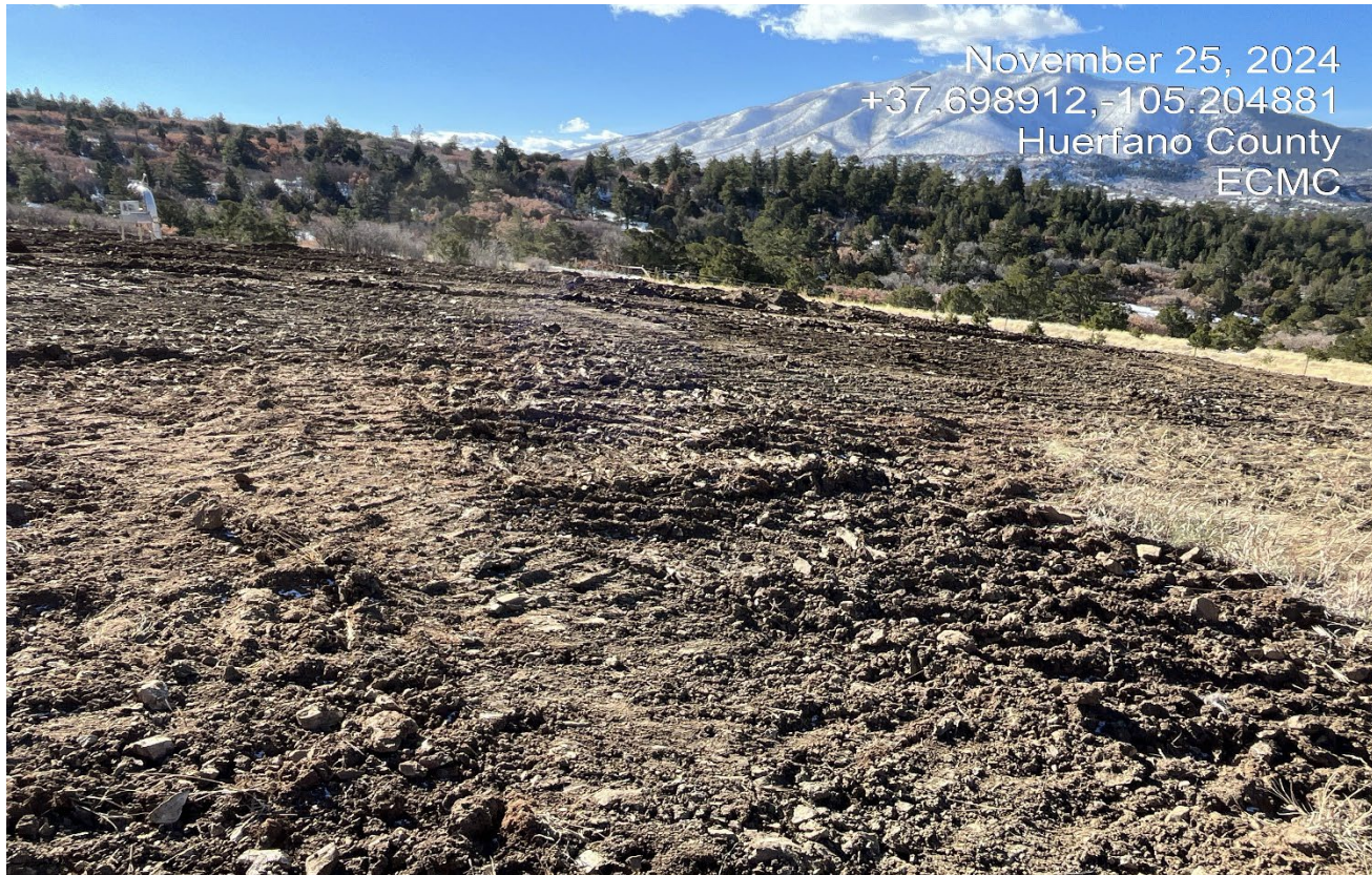
Photo 3. Facing southwest at the location. There appears to be more material in this area that needs to be pushed up toward the cu slope.
