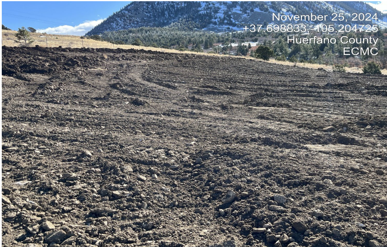
Photo 5. Facing southeast at the location. This area appears to need more material to match surrounding contours. Recontouring is still in process.
