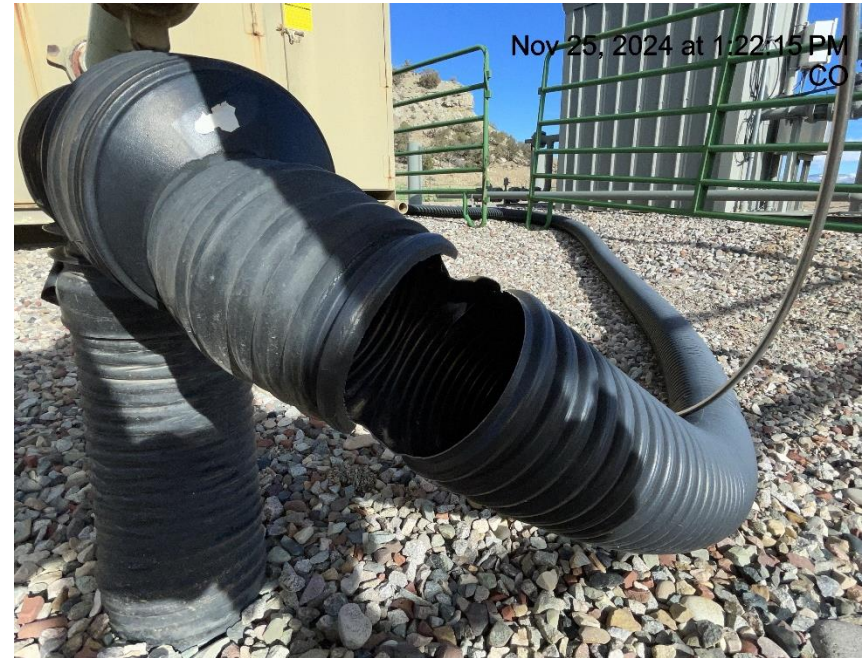
Photo # 1709 Flowline heating insulation damaged/wildlife hazard/available for entry by wildlife
