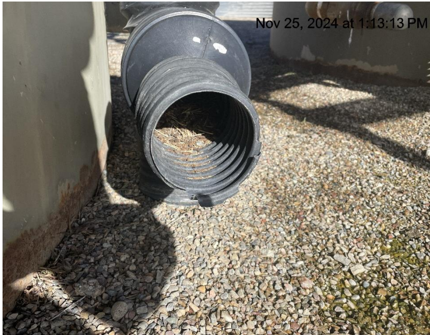
Photo # 1708 Flowline heating insulation open ended /wildlife hazard/available for entry by wildlife
