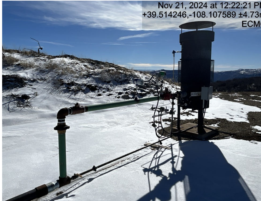
ECD flow line metered
