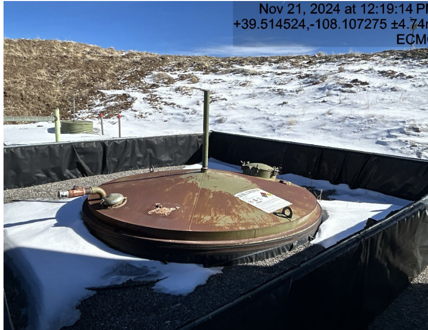
Condensate tank venting
