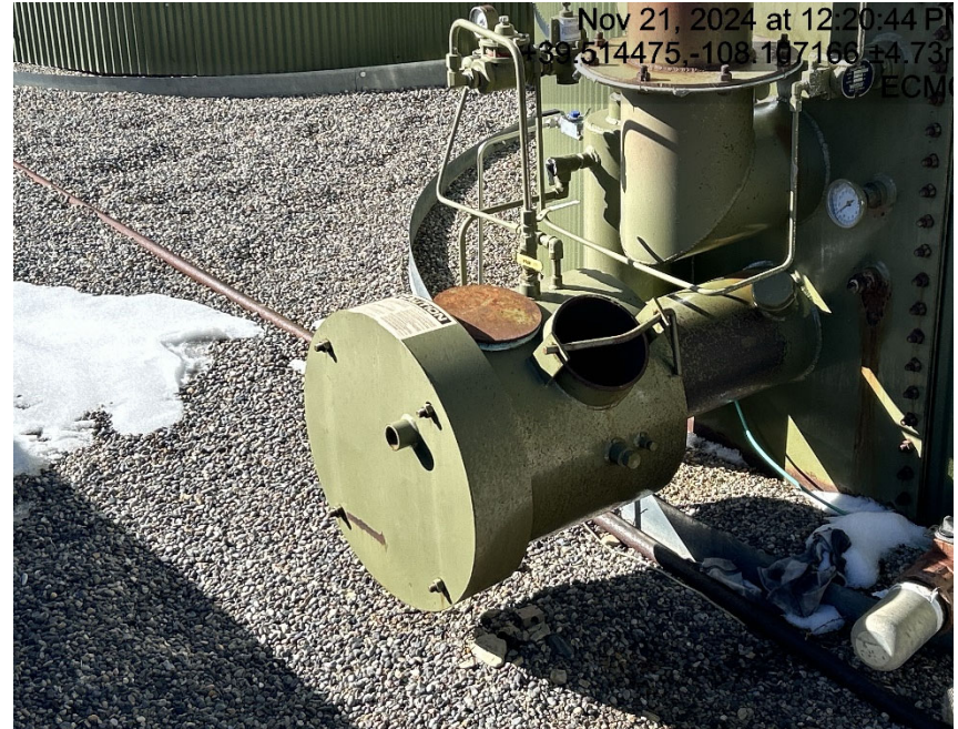
Open tank burner open for wildlife to enter
