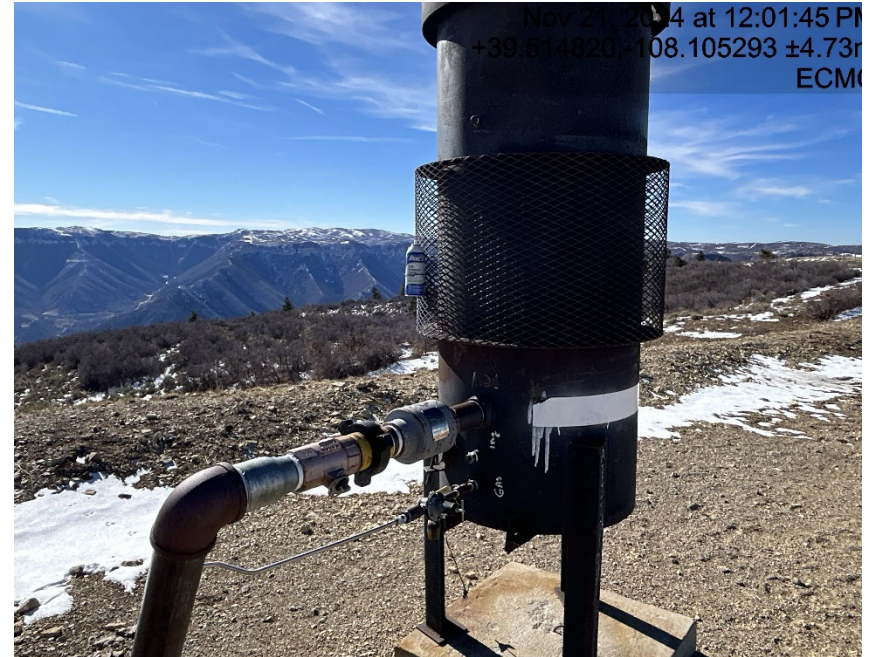
No evidence of metering on flow line
