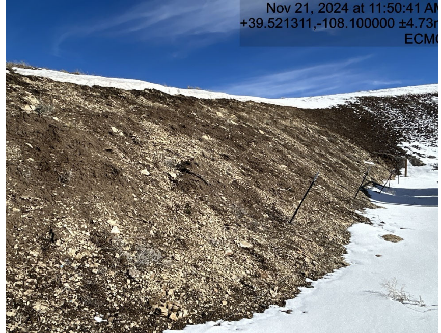
Cut slope shows some signs of lack of stablization
