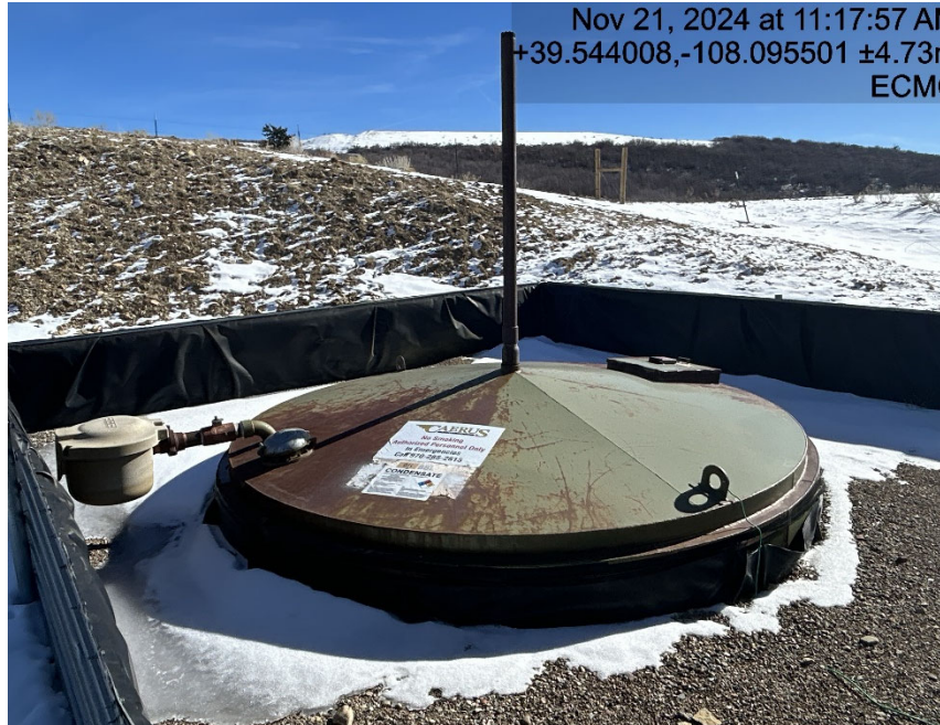
Condensate tank venting
