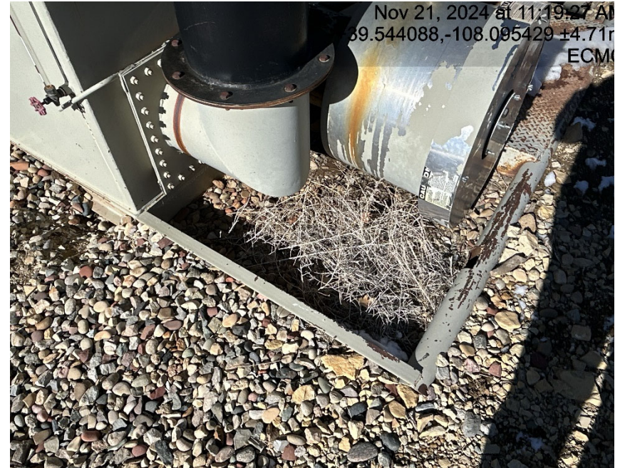
Weeds under burner assembly
