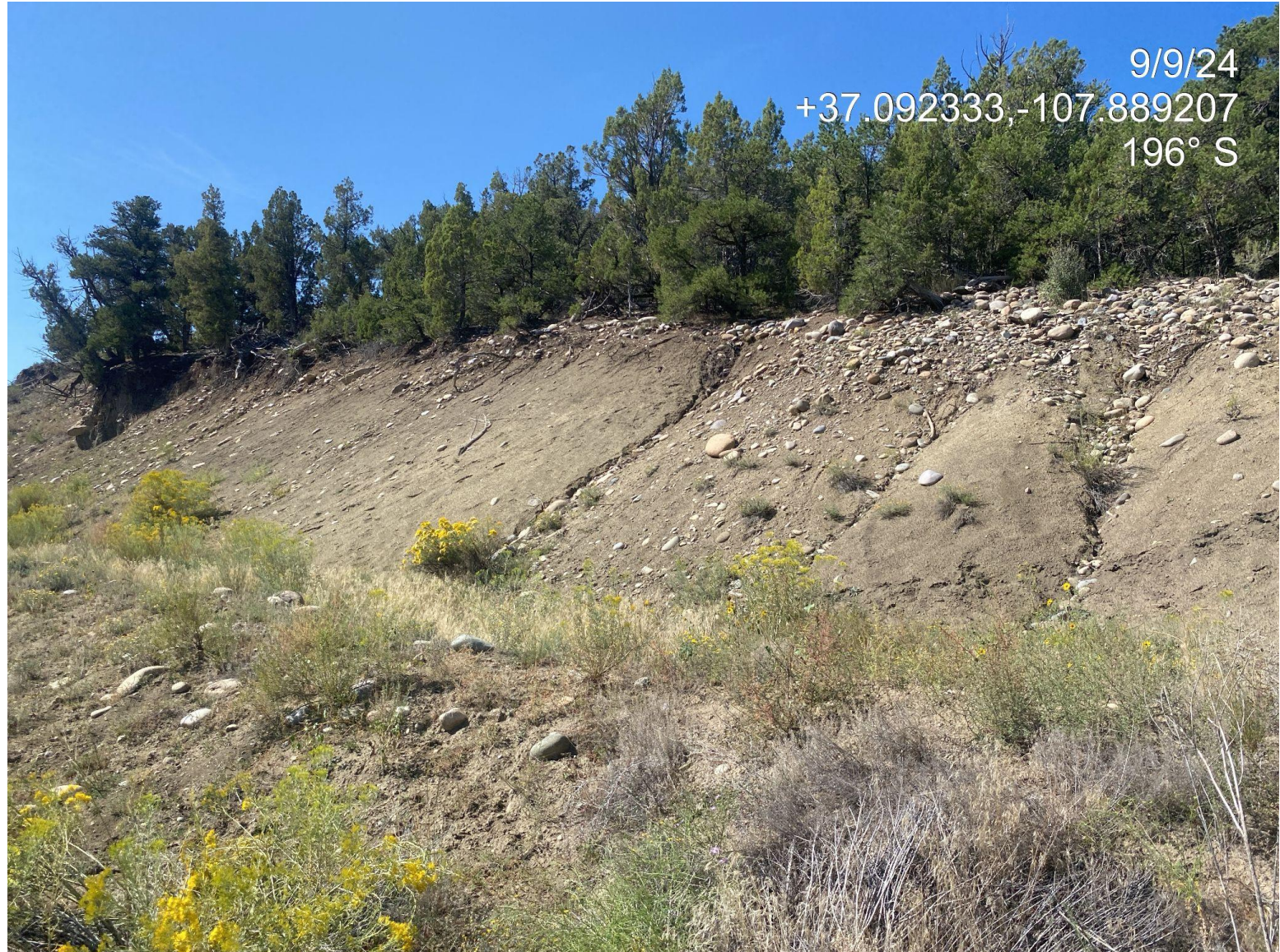
Photo 2. View of western cut slope area that remains with bare soil and minimal vegetation.
