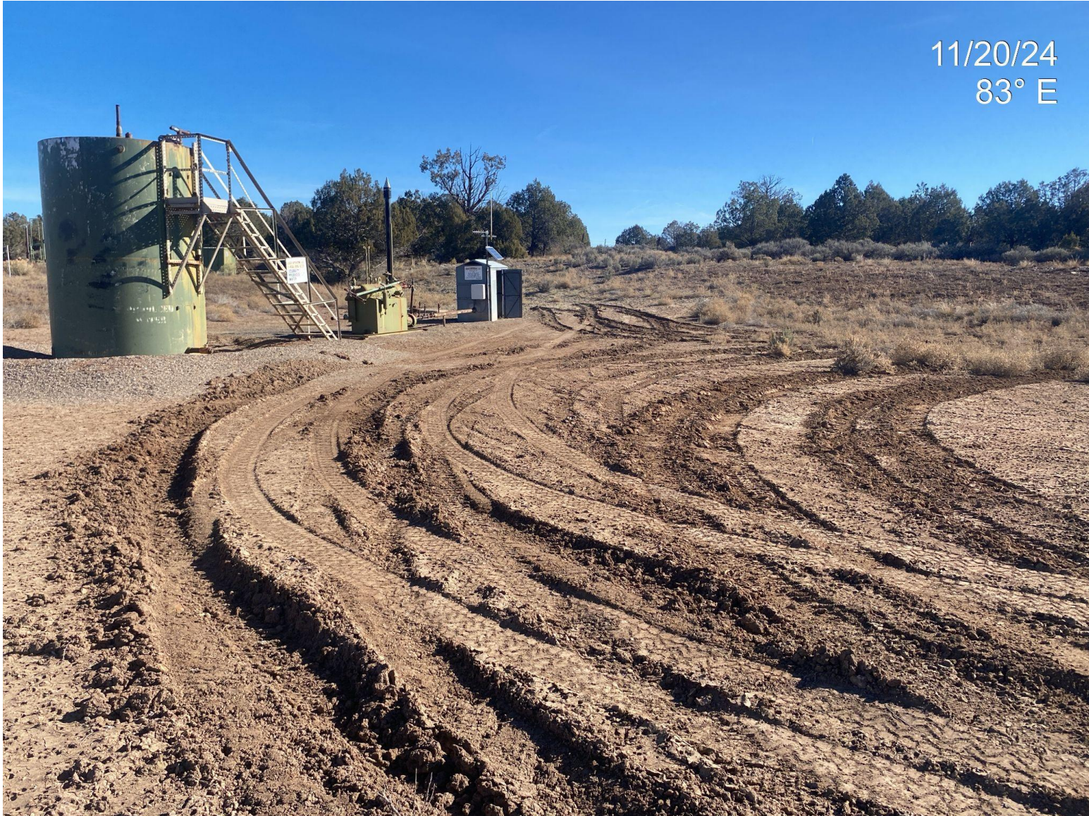
Photo 3. Rutting on active pad. Additional stabilization/grading needed. Note: unused equipment remains on location.
