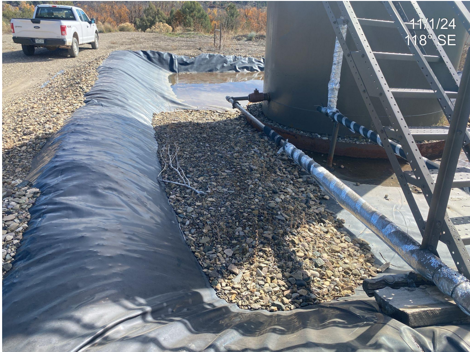
Photo 2. Gravel in produced water tank secondary containment which is affecting overall capacity/volume.
