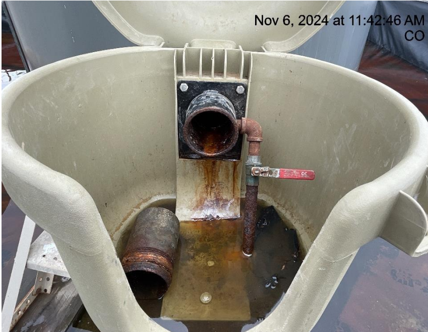
Photo # 9420 From inspection 708904982 conducted on 11/06/2024 - Open ended load line
