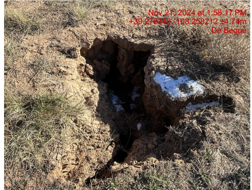
Photo # 9621 Subsidence in multiple areas on east side of location is also a wildlife/personnel safety hazard
