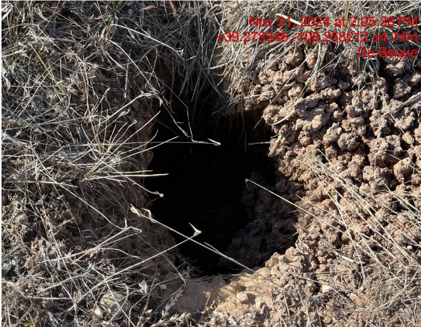
Photo # 9644 Subsidence in multiple areas on east side of location is also a wildlife/personnel safety hazard
