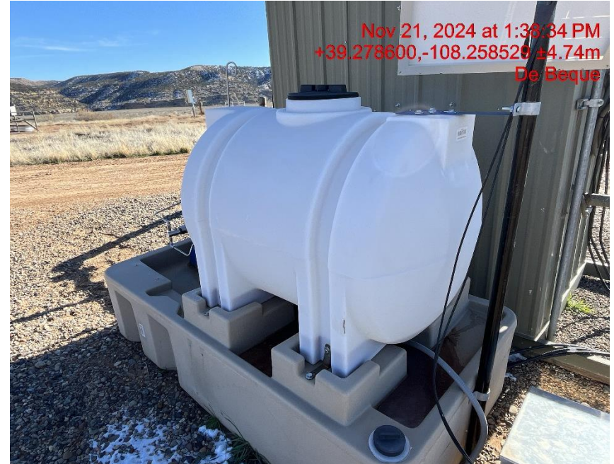
Photo # 9601 Chemical tank is not labeled
