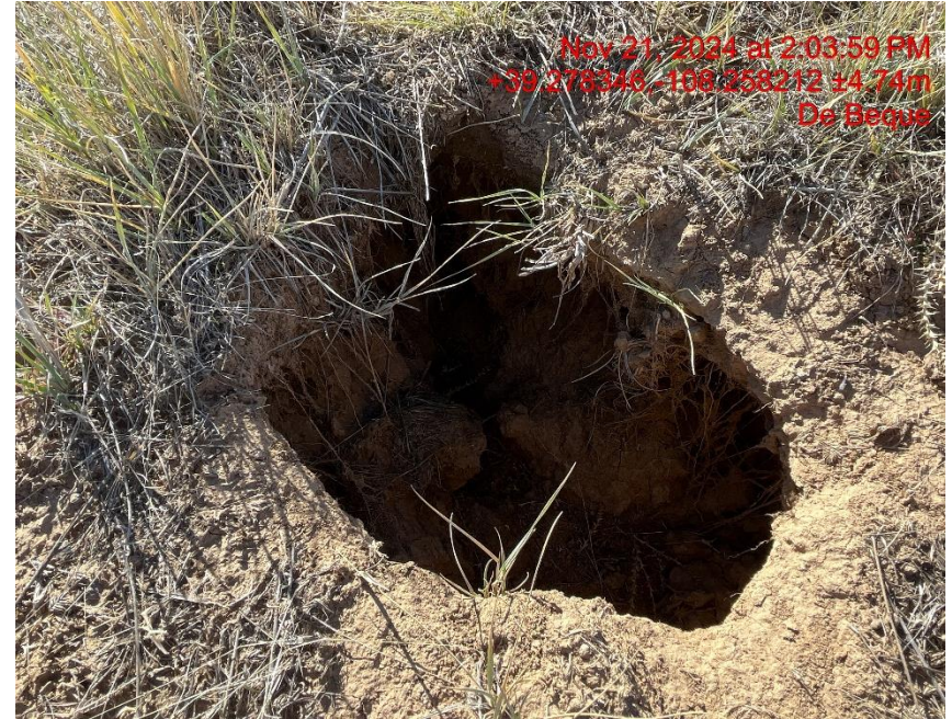
Photo # 9639 Subsidence in multiple areas on east side of location is also a wildlife/personnel safety hazard
