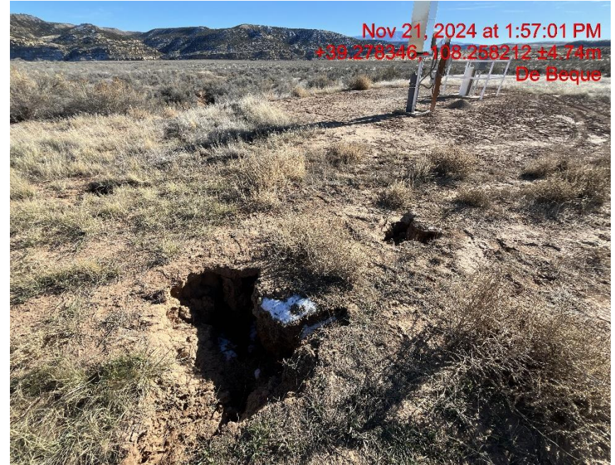
Photo # 9618 Subsidence in multiple areas on east side of location is also a wildlife/personnel safety hazard
