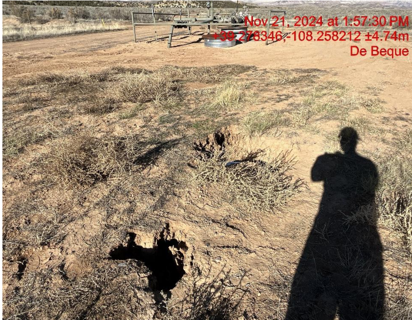
Photo # 9620 Subsidence in multiple areas on east side of location is also a wildlife/personnel safety hazard
