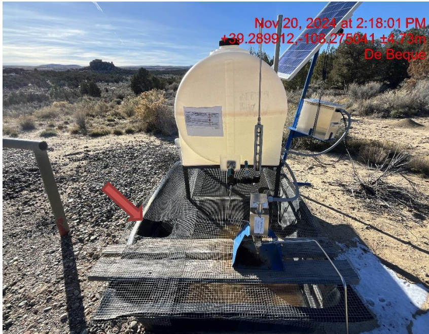
Photo # 9391 Wildlife protection for chemical containment needs maintenance/screen is damaged and open to wildlife
