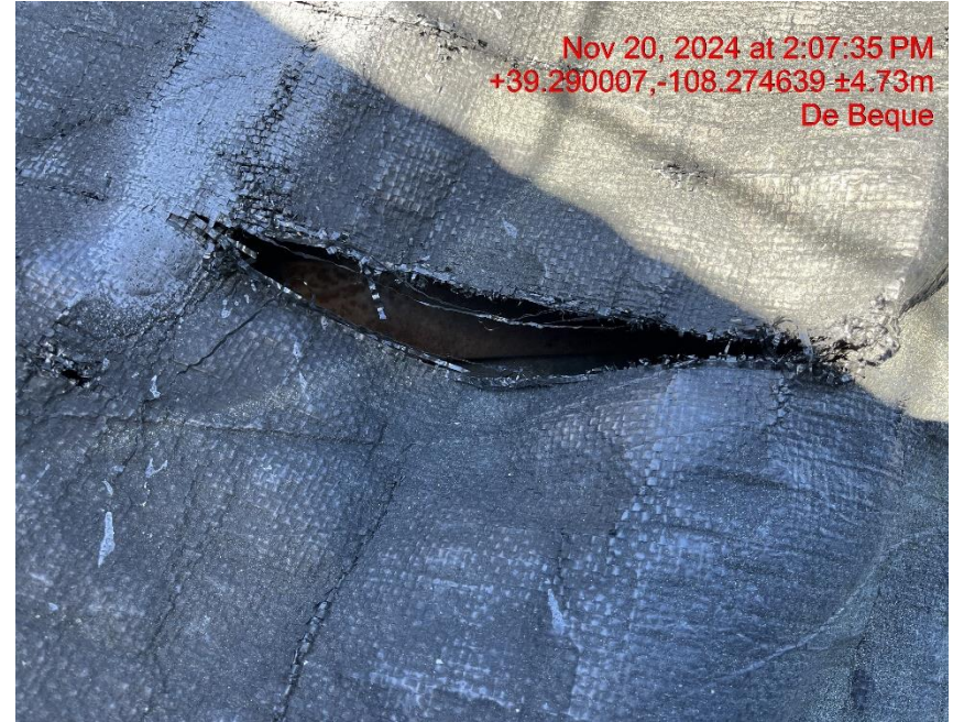
Photo # 9382 Multiple holes and tears in secondary containment liner/liner needs maintenance, also the liner is deteriorating and lacks integrity
