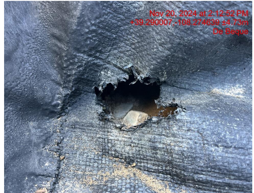
Photo # 9387 Multiple holes and tears in secondary containment liner/liner needs maintenance, also the liner is deteriorating and lacks integrity
