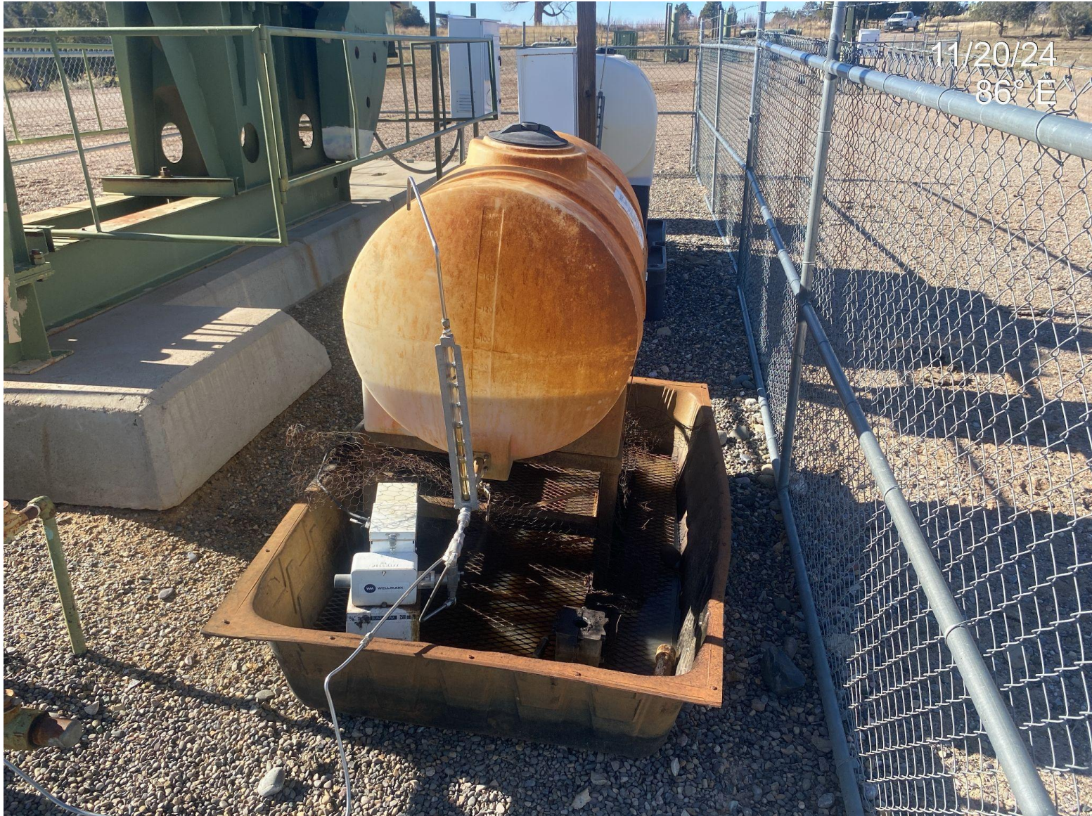
Photo 4. Wildlife BMP netting/wiring at chemical container secondary containment is damaged and no longer functioning.
