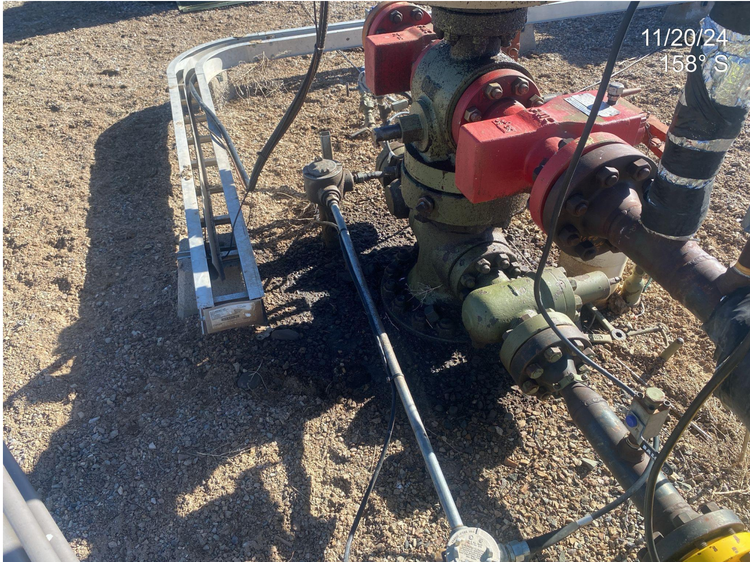
Photo 5. Impacted surface material observed at well head.
