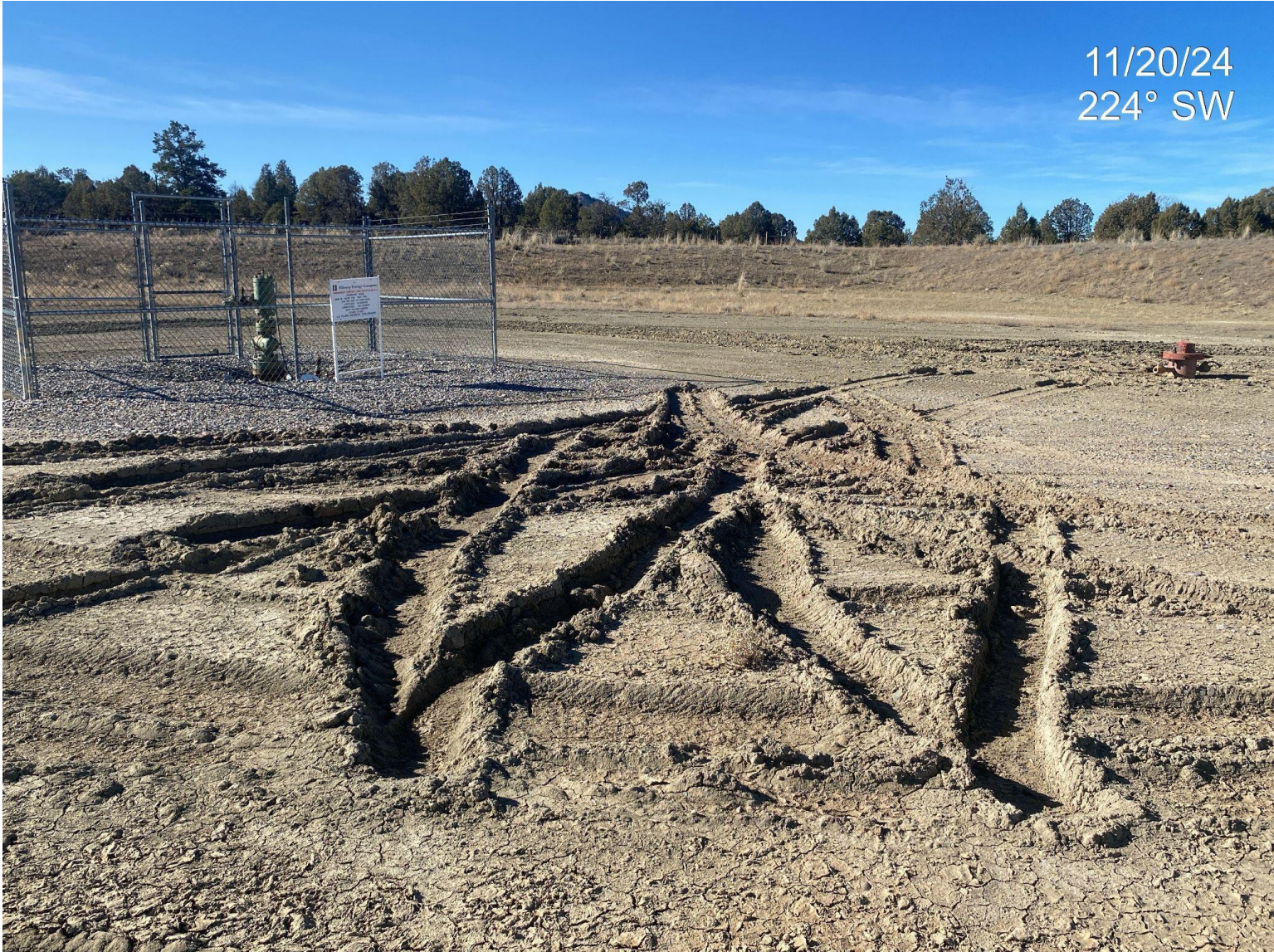
Photo 4. Rutting occurring on active pad.
