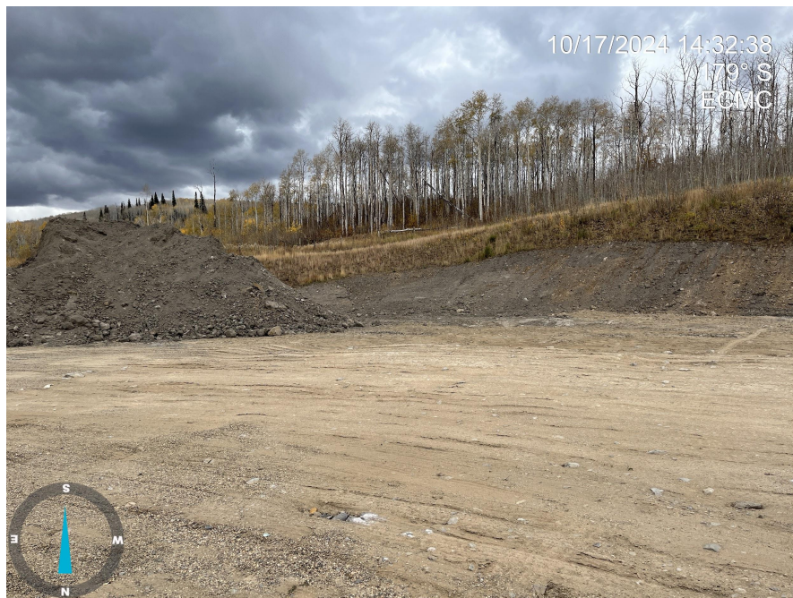
Photo 1. Photo taken from western portion of Location, facing south. Photo illustrates that the cuttings pile is missing containment measures. At the time of inspection, cuttings were in process of being removed from the Location.
