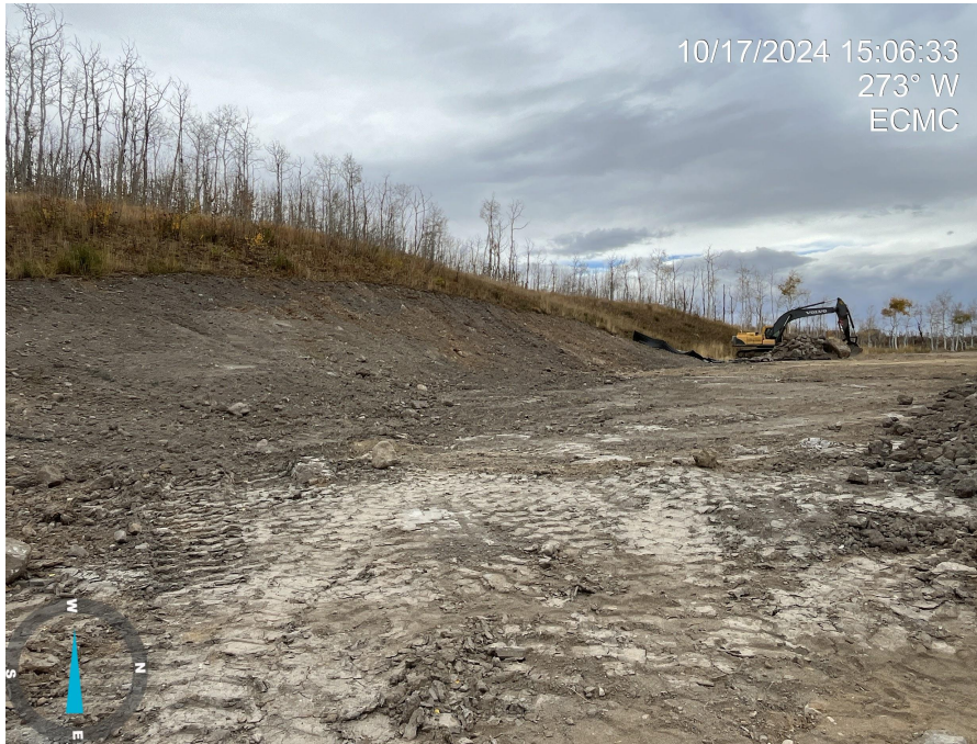
Photo 3. Photo taken from southern portion of working pad surface, facing west. Photo illustrates inadequate/missing secondary containment measures around cuttings pile.
