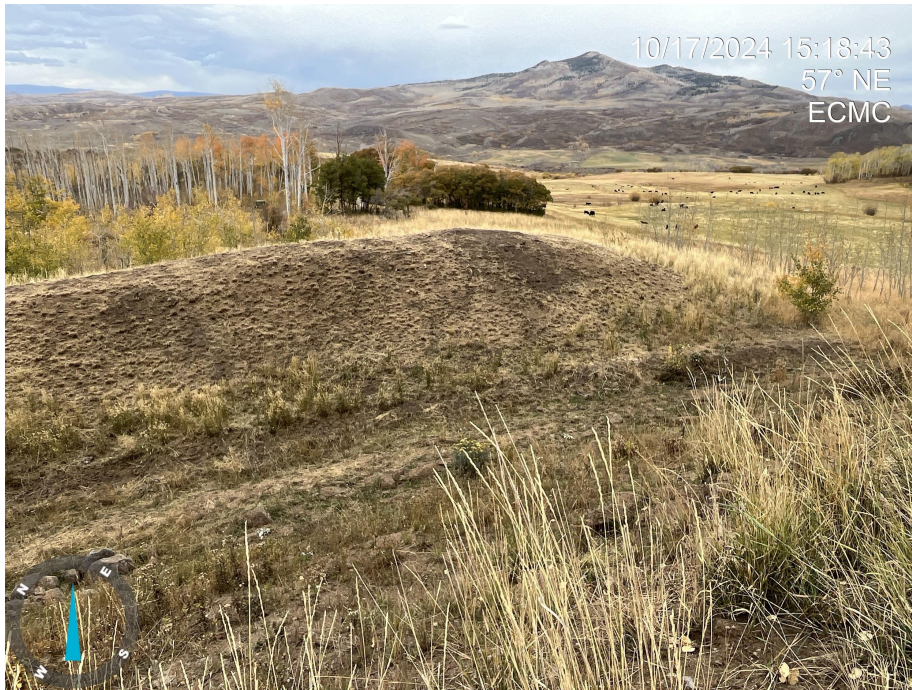
Photo 11. Photo taken of the topsoil stockpile. BMPs (hydromulch) have been implemented to reduce slope erosion and degradation.
