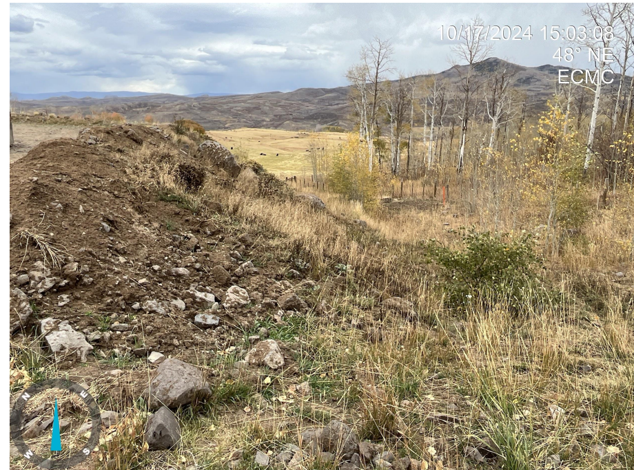
Photo 12. Photo taken of eastern fill slope area, facing northeast. BMPs (hydromulch) have been implemented to reduce slope erosion and degradation.
