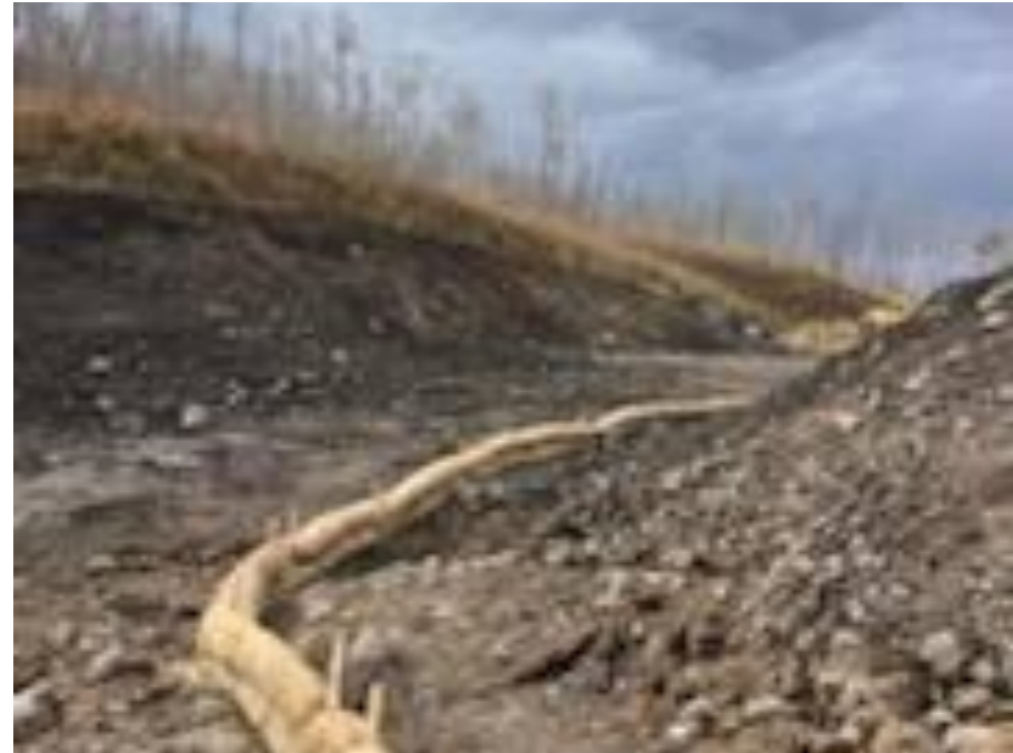
Photo 4. On 10/18/2024, photo submitted by Operator. Photo illustrates adequate containment measures implemented around the cuttings pile 10/18/24.
