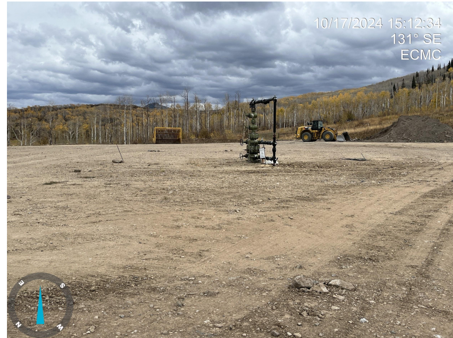
Photo 14. Photo taken from western edge of Location, facing southeast. Photo illustrates that all risers and flowline equipment have been removed.
