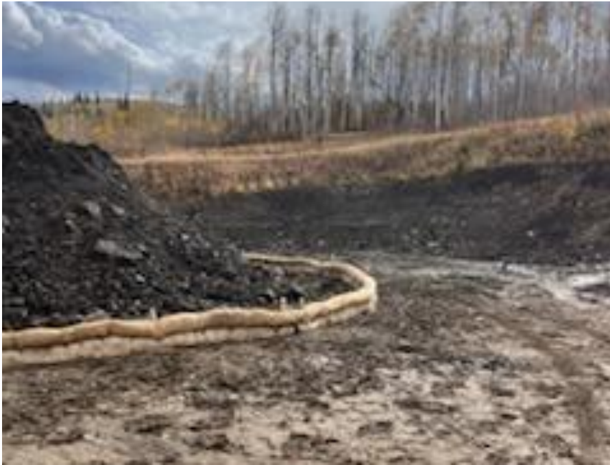
Photo 5. On 10/18/2024, photo submitted by Operator. Photo illustrates adequate containment measures implemented 10/18/24. Adequate containment measures implemented 10/18/24.
