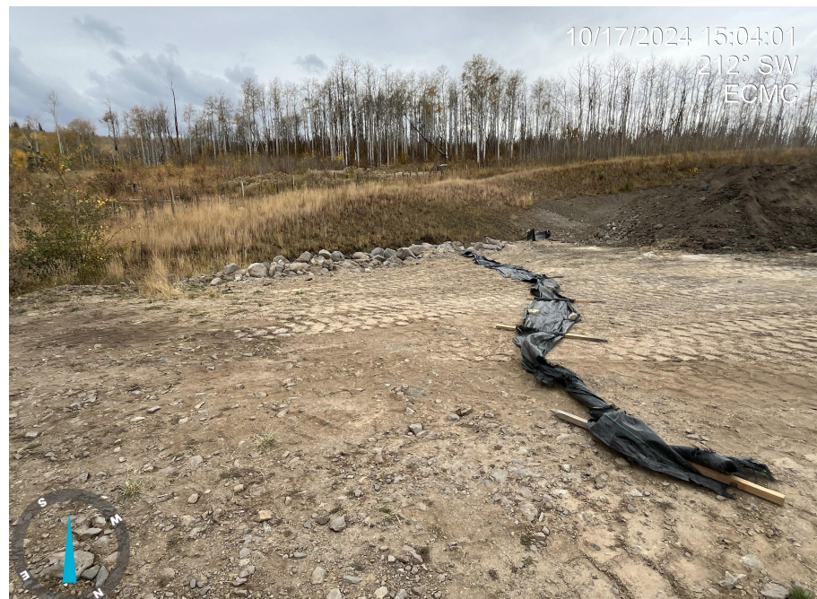
Photo 2. Photo taken from southern portion of Location, facing southwest. Operator previously implemented silt fence to protect offsite movement of E&P waste. BMP was not properly maintained and inadequate in containing E&P waste. Operator indicated that they removed silt fence 10/18/2024.
