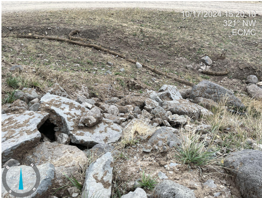
Photo 7. Photo taken of northern fill slope, illustrating the stormwater outlet. Geotextile lining in conjunction with multiangular rip-rap material has been implemented at the outlet on the north end of the Location.
