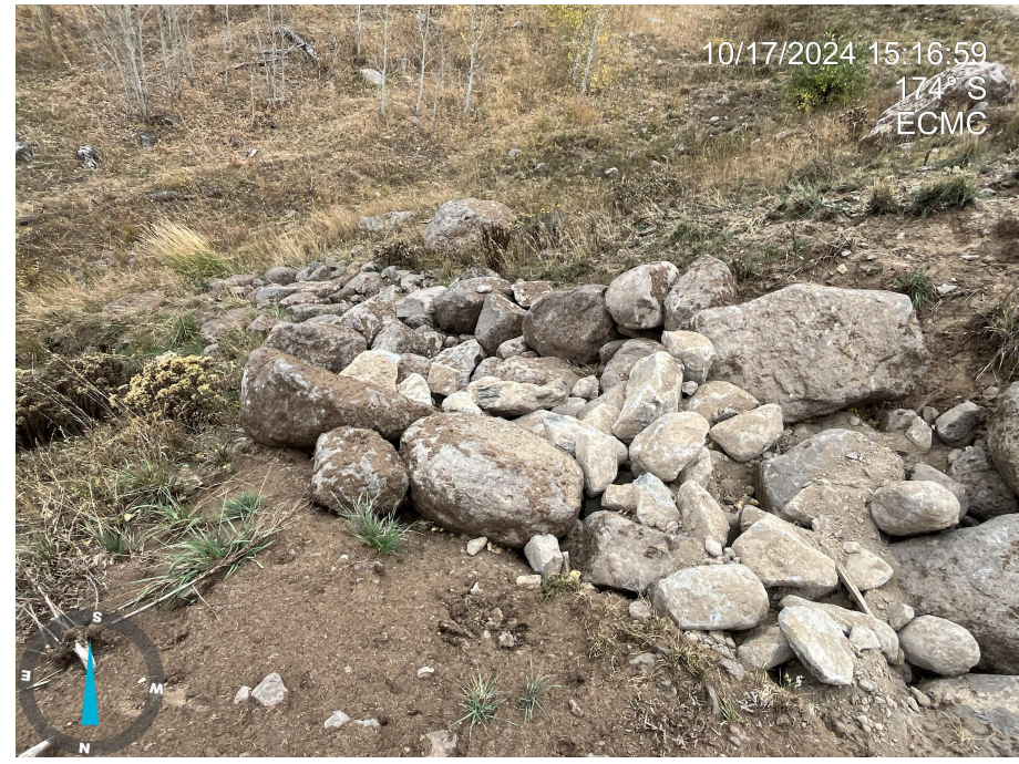
Photo 8. Photo taken on eastern edge of Location, illustrating the stormwater outlet has been lined with a geotextile material in conjunction with multiangular rip-rap.
